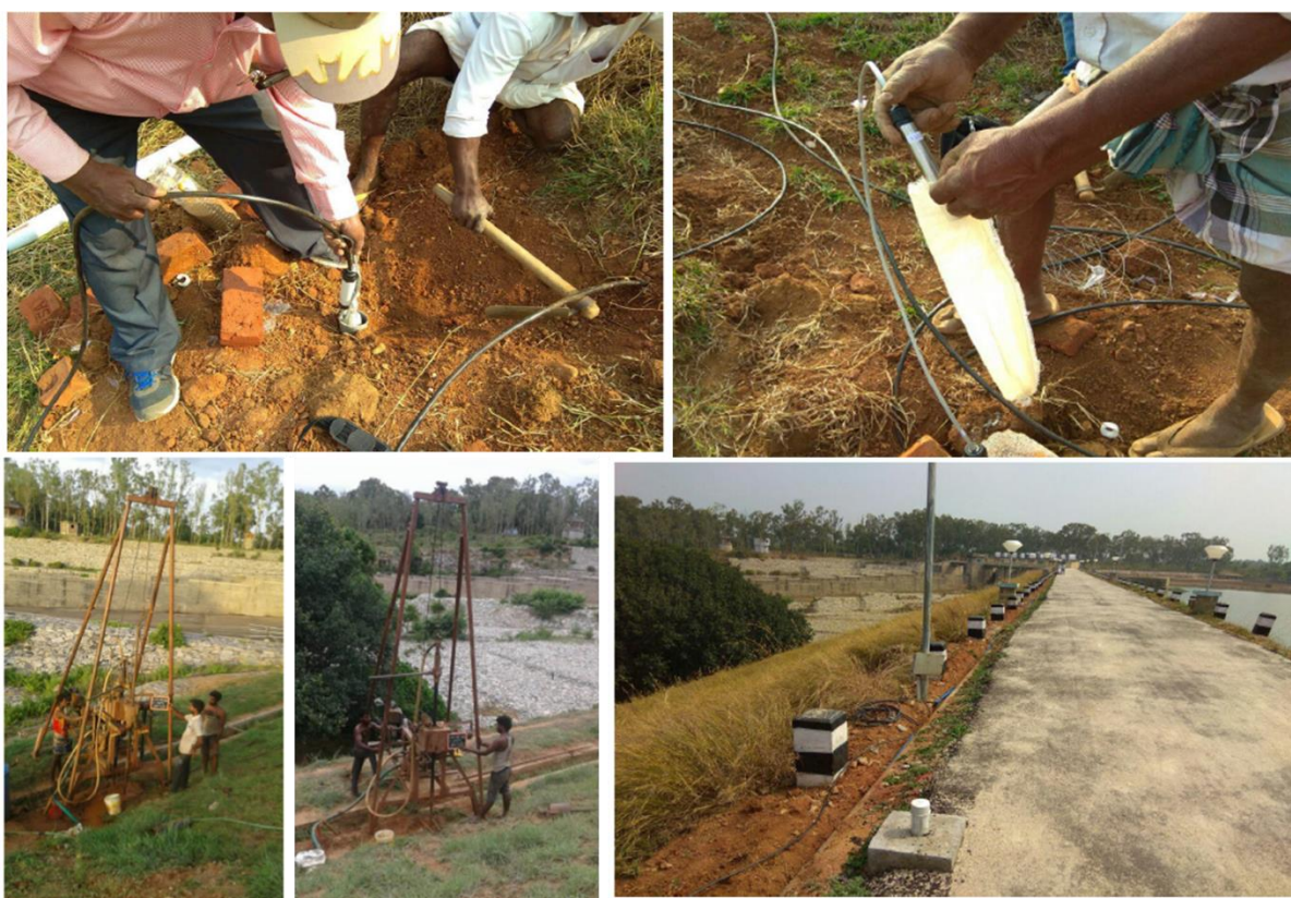
Figure B.4.- Installation of Pizometers in Embakment Dam.
