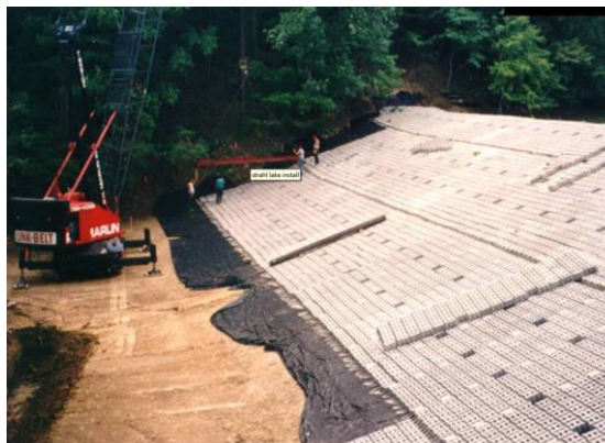
Figure 6.4.- Placement of cable-tied mats over a geotextile on the downstream face of Strahl Lake Dam, Indiana (Photo by Contech Construction Products, Inc.)
