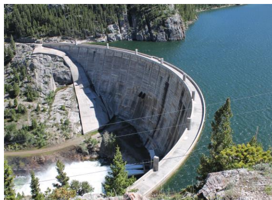
Figure 6.5.- Overflow Protection in abutments (Gipson Dam, US)
