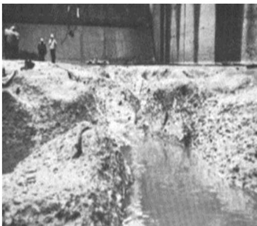
Figure 5-69: Severe damage by abrasion, bottom slab of stilling basin, Libby dam (USACE, 1980)
