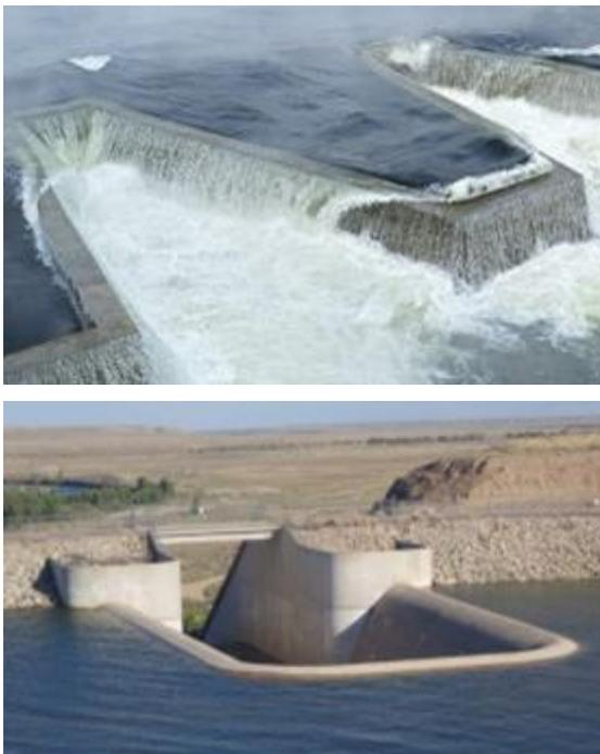
Figure 3-12: Service spillways. Control structure: bathtub or duck bill weir
