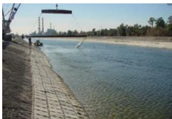
Figure 5-57: Articulated concrete blocks (ACB) as mattresses, bank protection in excavated channel
