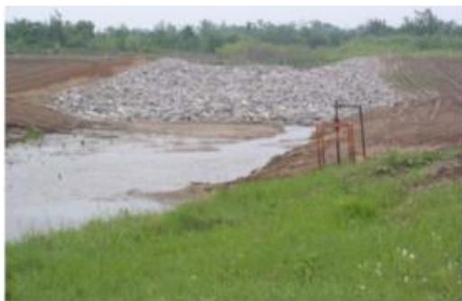
Figure 2-27: Rock chute spillway of Little Washla Site, USA.
