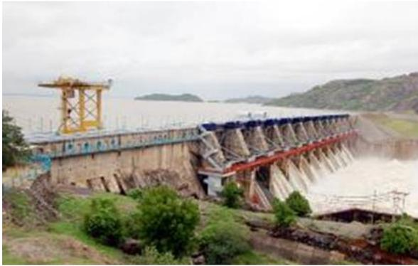
Figure 5-36: Dharoi dam, height 46 m, Solid Roller Bucket,  $Q = 21,662 \text{ m}^3/\text{s}$
