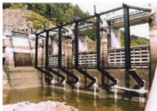
Figure 2-16: Spillway's Trash-racks.
