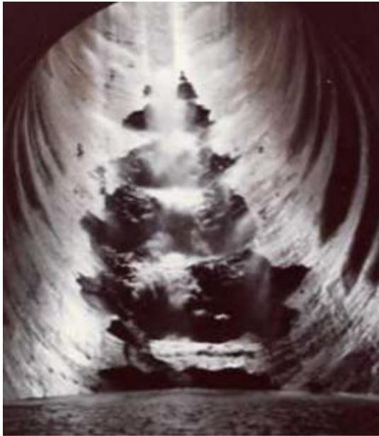
Figure 4-42: Cavitation in Tunnel Spillway of Glen Canyon Dam (USBR, 1983)
