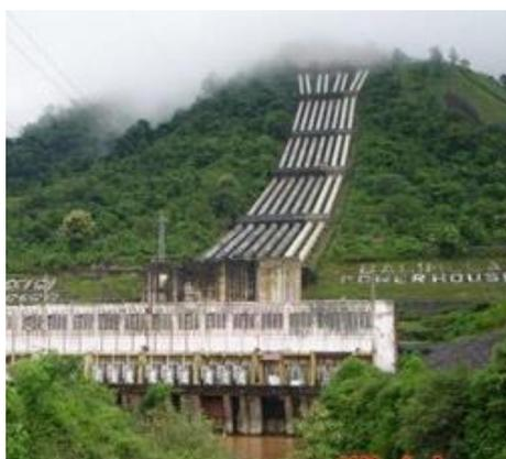
Figure 4-8: Penstock (8 no.) to Balimela Power House - Machkund-Sileru River (Odisha Hydro Power Corporation Ltd)
