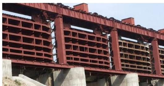
Figure 4-27: Stoplog gates (Shree Shakti Eng.)
