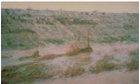
Figure 2-26: : Vegetated embankment experienced overtopping flow.
