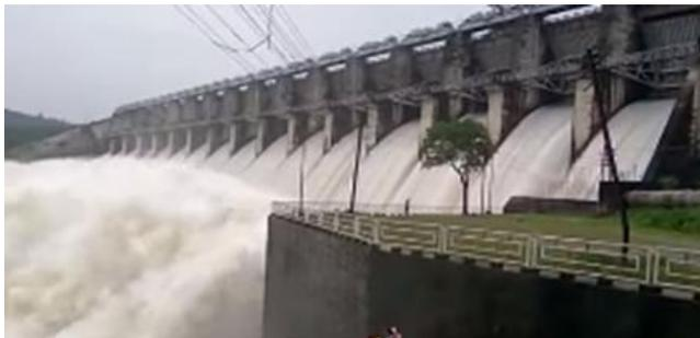
Figure 5-38: Kadana dam, height 66 m, Solid Roller Bucket,  $Q = 49,497 \text{ m}^3/\text{s}$
