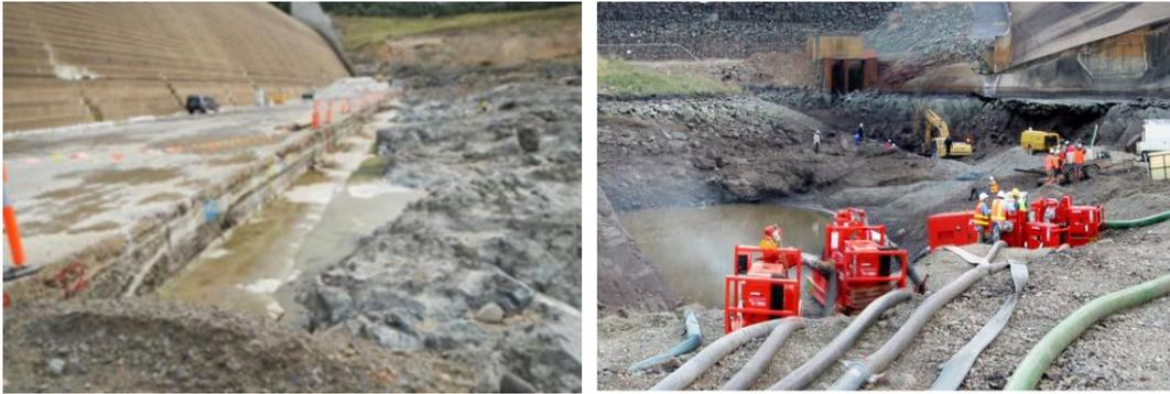
Figure 5-84: Erosion after a season of floods, Paradise and Borumba dams, Australia (Bollaert, et al, 2016 and 2014)
