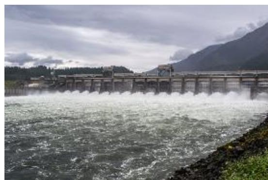
Figure 5-60: Flow pattern at exit channel in a low head spillway
