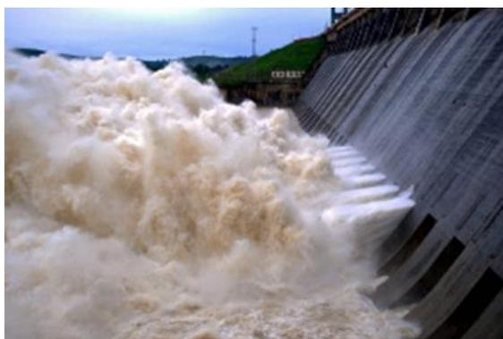
Figure 3-28: Typical bottom outlet in overflow dam section
