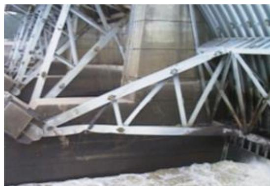
Figure 3-148: Failure of a strut arm of a radial gate by impact
