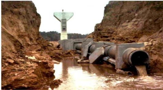
Figure 4-47: Internal erosion around conduit in embankment dam
