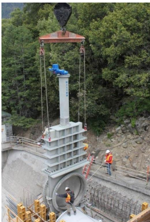
Figure 4-29: B A Hilton Throttling Knife Gate Valve at a California dam project (Hilton, 2015)
