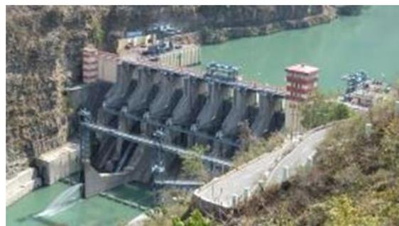
Figure 5-33: Ichari dam, height 59 m, Slotted Roller Bucket, Q= 13,500 m<sup>3</sup>/s
