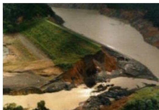
Overflowing of chute's walls, erosion of abutment, undermining of chute, head cutting and collapse of spillway (see Case Study in Appendix).
