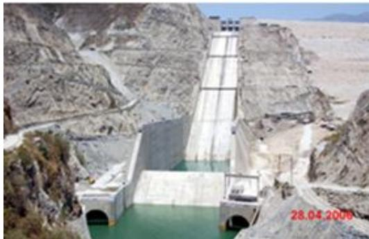
Figure 5-44: Tehri dam, India, surface spillway and outlet of right bank tunnels.
