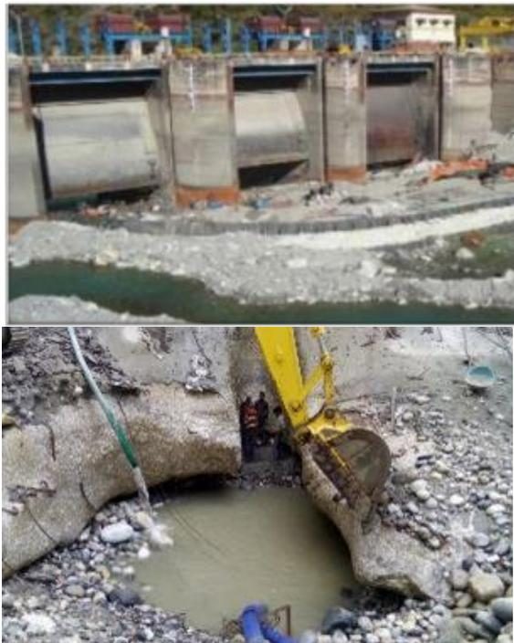
Figure 5-71: Severe damage by abrasion in terminal structure, Maneri dam, India (CWC)
