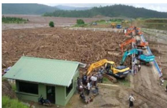
Figure 2-11: Clearing a blocked dam.
