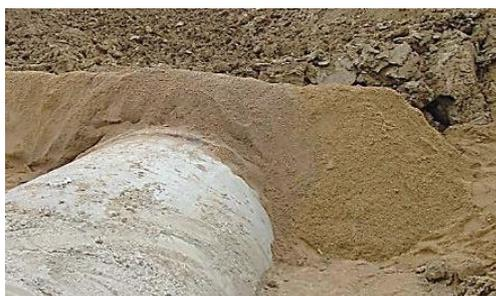
Figure 4-53: Typical configuration for a filter diaphragm. (FEMA, 2005)
