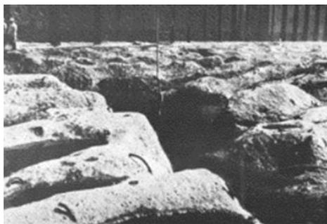
Figure 5-77: Cavitation at bottom slab for  $V = 48$  m/s (3 m deep), Dworshak dam (USACE, 1980)
