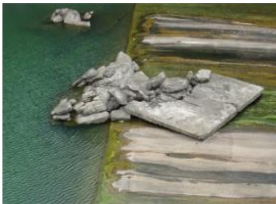
Figure 5-80: Moved slabs by high velocity flow, Bhama Askhed dam, India
