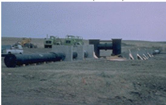
Figure 4-61: Antiseep collars in outlet conduit during construction. (ASDSO)
