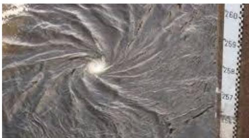
Figure 4-37: Guri Dam. Vortex at intake hydropower plant (EDELCA, 2001)
