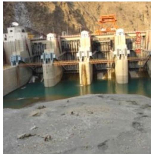
Figure 5-43: Bottom outlet spillway. Chamera II Dam, India (Bhajantri et al, CWPRS, Pune)
