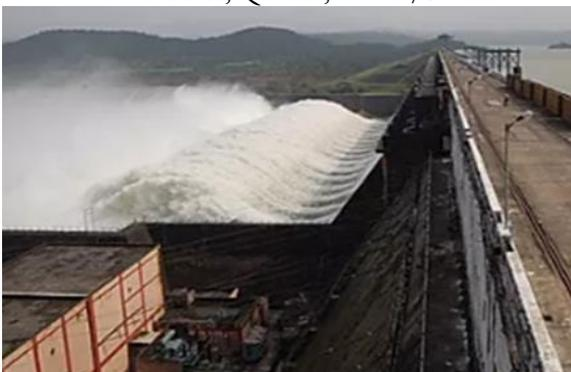
Figure 5-40: Ukai dam, height 105 m, Flip Bucket,  $Q = 42,269 \text{ m}^3/\text{s}$
