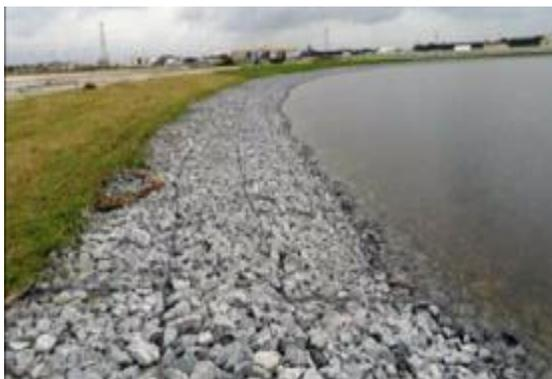
Figure 5-58: Gabions, Reno mattresses, bank protection in excavated channel
