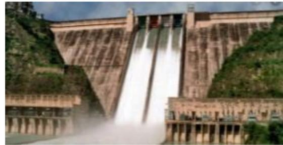
Concrete Gravity dam, 226 m high. Spillway Stilling basin was damaged (see case study in "Manual on Rehabilitation of Large Dams")
