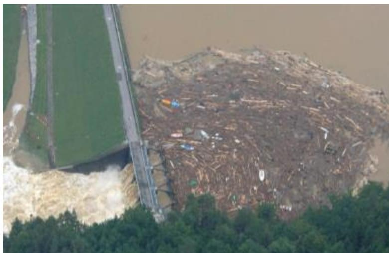
Figure 2-5: Floating debris in front of Thurnberg Dam Spillway, Austria, during the extreme flood of 2002
