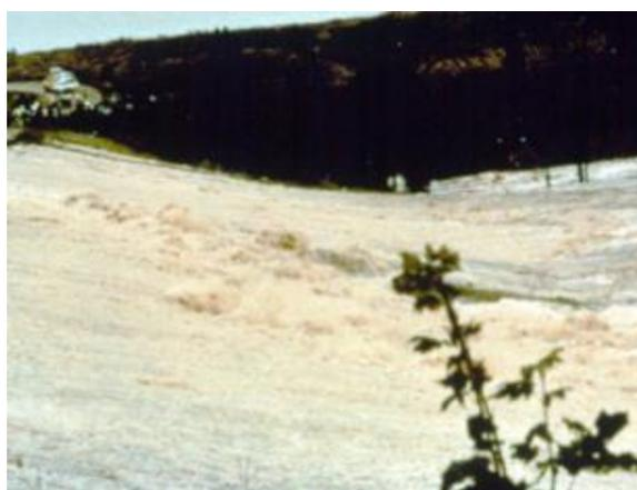
Figure 2-22: Overflow on an Embankment dam.
