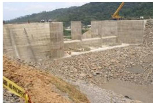
Figure 2-37: Approach Channel for the ungated El Guapo Spillway Dam, Venezuela, (Photo A Marcano)
