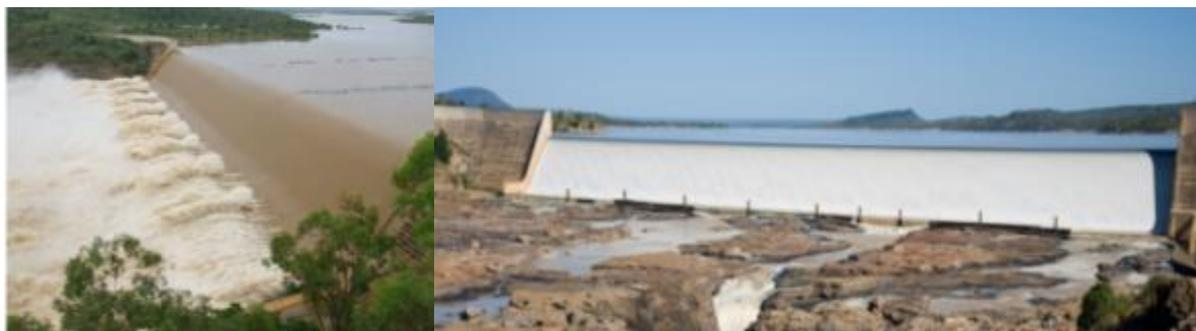
Figure 3-10: Service spillways. Control structure: free discharge, straight shaped crest. Burdekin Falls Dam; Australia. Spillway Capacity: 64,600 m<sup>3</sup>/s
