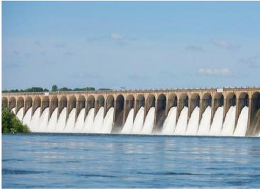
Figure 3-25: Wilson Dam, Alabama. Orifice spillway; flow is controlled by 58 gates (USA, 1926).
