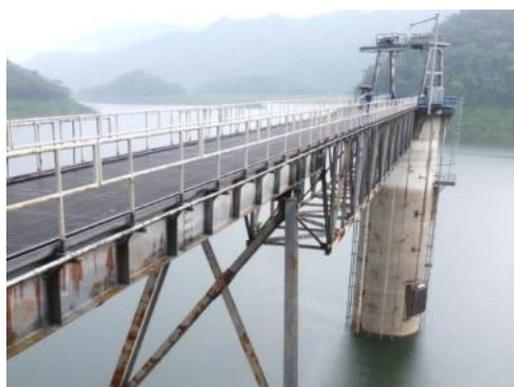
Figure 4-57: 109 m high Tower Intake Turimiquire Dam
