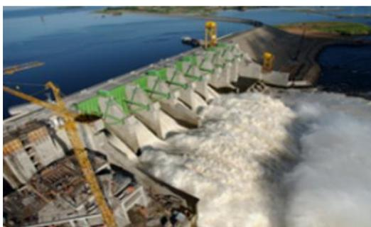
Figure 5-7: Energy dissipation by impact flip bucket (EDALCA, Venezuela)
