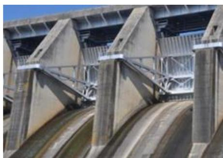
Figure 3-117: Typical Radial (Tainter) gate (USACE)
