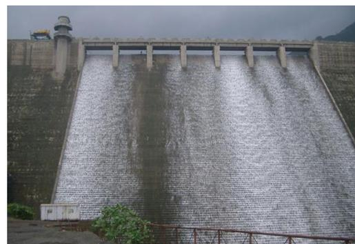
Figure 3-102: Ghatghar Lower Dam. First RCC dam in India; 14 years in operation (Patel Engineering)
