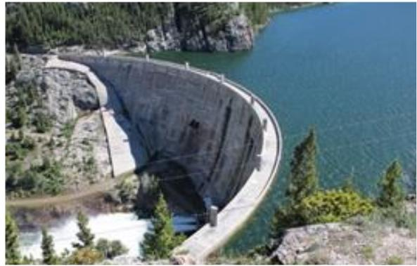
Figure 2-32: Photo showing Gibson dam and right abutment protection concrete
