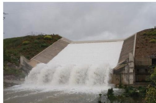
Figure 3-114: Hydraulic 3D model and stepped spillway; precast concrete blocks and trapezoidal section; Barriga Sam (Moran and Toledo, 2006)
