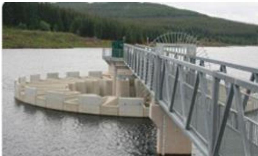
Figure 3-70: PKW on a Morning Glory weir to increase spillway capacity. Our Black Esk Dam (USA).
