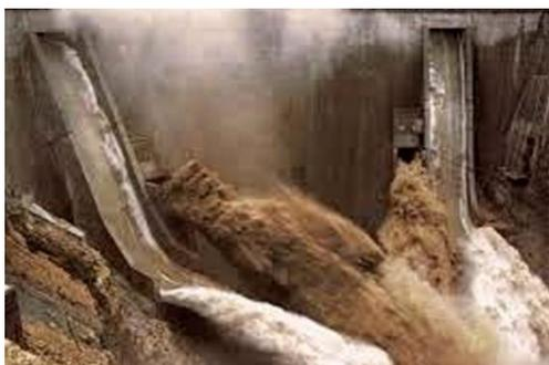
Figure 4-11: Sediment removing at Jiroft Dam – Iran(www.entura.com.au)
