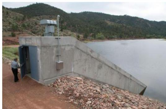
Figure 4-24: Inclined Intake Tower Nichols Reservoir, USA. (Albuquerque Journal; 2014)
