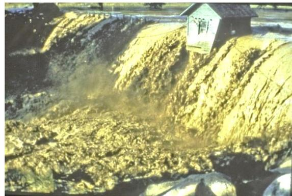
Figure 4-65: Cascade Dam overtopping. July 15th 1982 (ASDSO)
