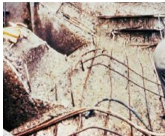
Figure 5-70: Severe damage due to abrasion, loss of baffle blocks (FEMA, 2010)
