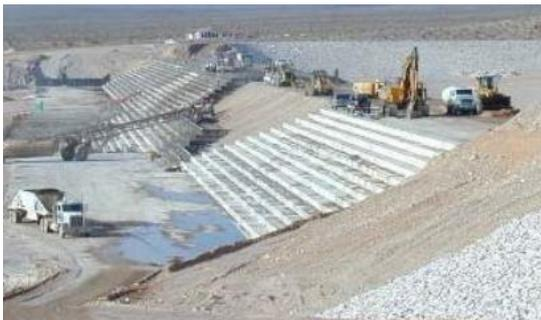
Figure 3-111: Construction of steeped spillway on an earth dam; Las Vegas, USA. (USACE and H. Chanson, 2009)
