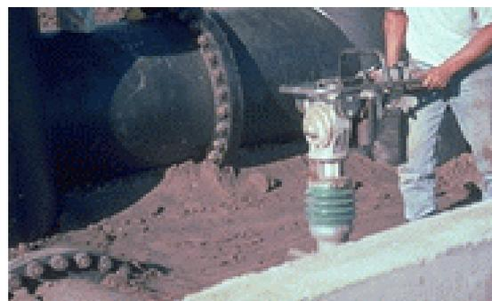
Figure 4-62: Manual compaction around conduit (ASDSO)
