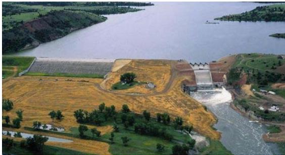
Figure 3-103: Tongue River Dam, USA. Two spillways: service (right) and auxiliary stepped chute (left) (FEMA, 2014)
