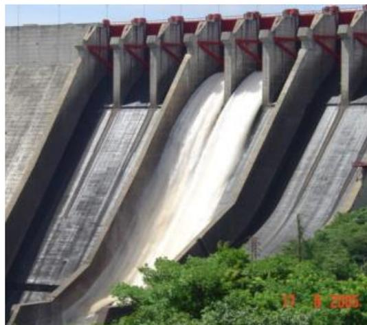
Figure 3-17: Service Spillways Chutes
