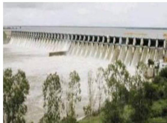
Very large spillway; radial gates, composite dam, 56.4 m high, 18,010 m<sup>3</sup>/s
