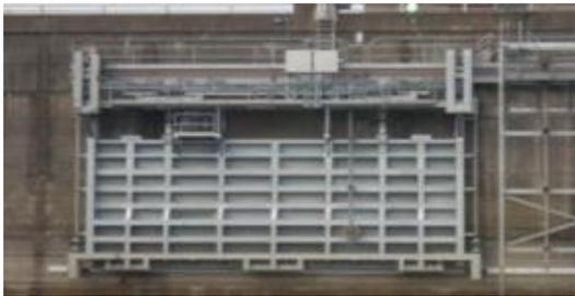
Figure 3-124: Typical installation of bulkhead gate (USACE)
