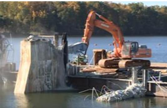
Figure 3-54: Townhead dam. Labyrinth weir. Phases of construction and demolition of old spillway(Schnabel Engineering)
