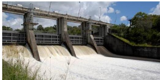
Figure 4-26: Vertical Lift Gates at Leslie Harrison Dam (Australia) (Shree Shakti Eng.)
