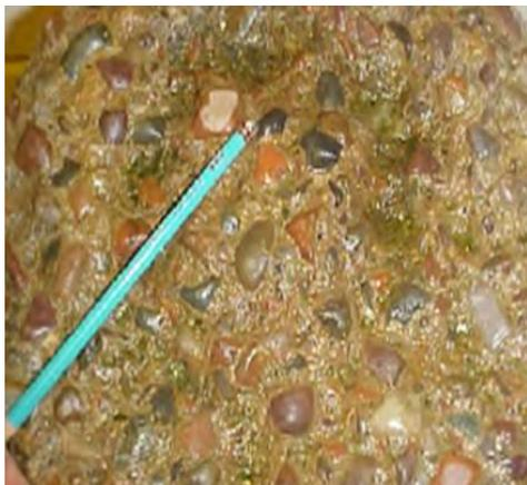
Figure 5-67: Incipient abrasion damage of concrete surface (FEMA, 2010)
