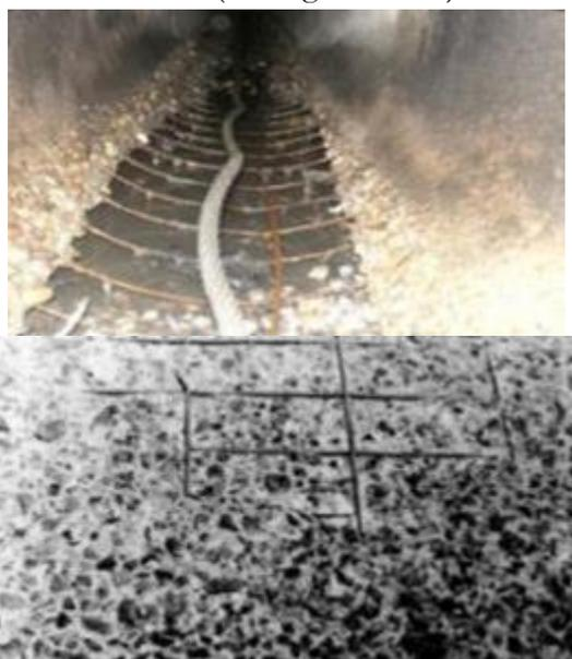
Loss of concrete element and cover of reinforcement bars are exposed to corrosion.
