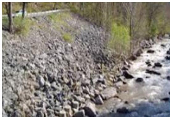
Figure 5-59: Rip-Rap, bank protection in natural channel
