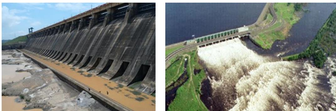
Figure 5-51: Combined Flip Bucket. Hirakud dam (India), surface spillway and sluices
