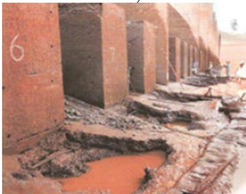
Figure 5-78: Cavitation damage downstream of chute blocks, Porto Combia dam, Brazil (ICOLD)
