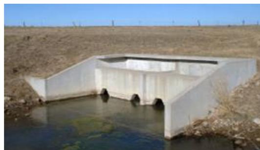
Figure 5-53: Impact basins (USBR Type VI), two structures placed side by side (FEMA, 2010)
