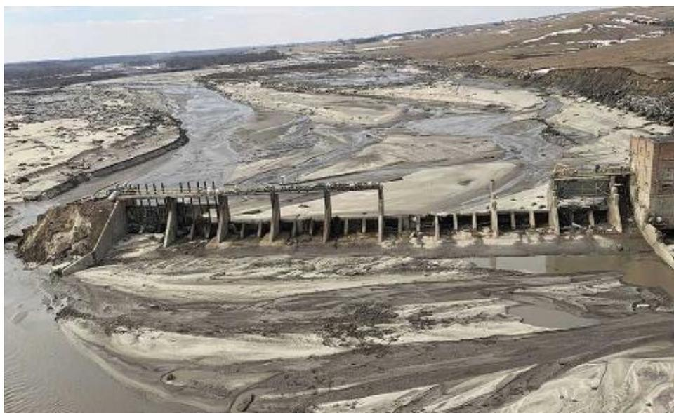
Figure 2-4: Spencer dam failure
