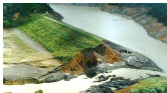
Figure 5-64: Hydraulic jump's swept out, head cutting erosion, loss of abutment with uncontrolled water release from reservoir, El Guapo dam, Venezuela
