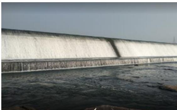
Figure 5-34: Damanganga dam, height 58.6 m, Solid Roller Bucket, Q=22,040 m<sup>3</sup>/s
