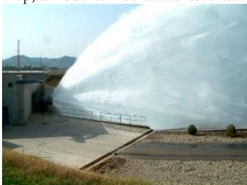
Figure 5-55: Fixed cone valve (Howell-Bunger) and typical discharge (diverged and hooded)
