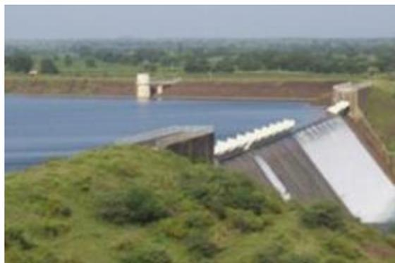
Spillway after tilting of 28 out of 66 fuse gates. Flood passing over the spillway -Storm of June 29/2005. (N. Solanki, SSEC).
