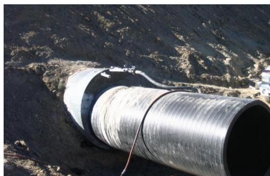
Figure 4-49: Annular space grouting Replace pipe in dam by a smaller diameter pipe (Mays construction)
