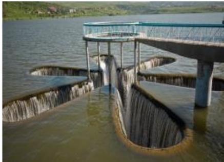
Figure 3-15: Service spillways. Control structure: drop inlet (Morning Glory) and special weir
