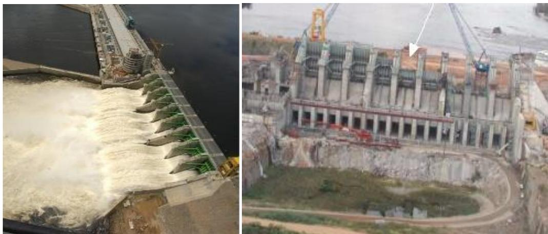
Figure 5-31: Excavated plunge pool, Caruachi dam, Venezuela;  $q = 200 \text{ m}^3/\text{s}/\text{m}$  (Marcano, 2000)
