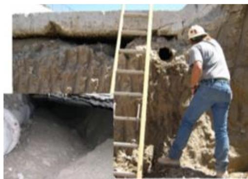
Figure 3-144: Failure of a chute's slab due to erosion. Hyrum Dam, USA (USBR, Trojanowski, 2005)
