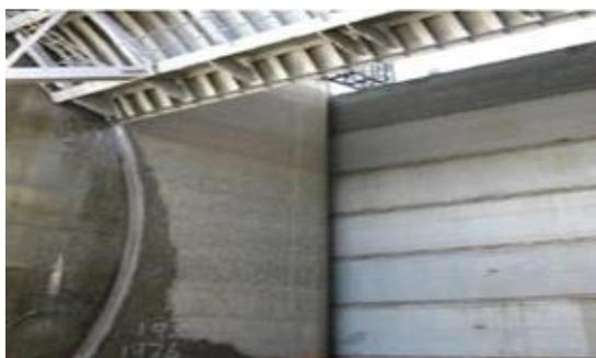
Figure 3-118: Typical installation of radial gate with stoplog (USACE)
