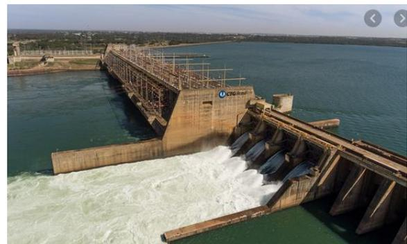
Figure 3-34: Jupia Hydroelectric Project, Brazil. 37 gates 6.6m (H)x 10m (W). Heat over sill=17m.  $Q = 44,400 \text{ m}^3/\text{s}$  (CESP).
