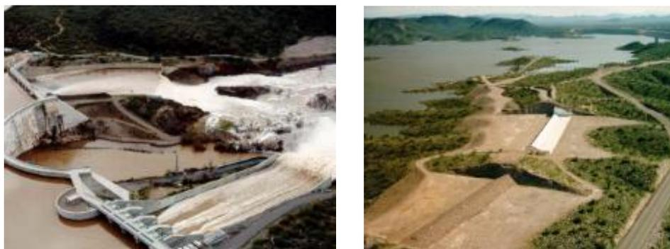
Figure 3-2: An illustration of service and auxiliary spillways located in dam and emergency spillway (fuse plug) located far away from the dam in reservoir rim
