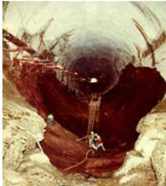
Figure 3-139: Cavitation damages plus erosion of rock and collapse of tunnel. Glen Canyon Dam, USA (USBR, ICOLD).
