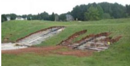
Y15 Dam (9.2 m high), Georgia, USA. IDF was  $\frac{1}{2}$  PMF. During flood, water depth on crest 0.37 m and unit discharge of  $0.4 \text{ m}^3/\text{s}/\text{m}$ . Soil and vegetation cover was locally washed out, but RCC was not damaged (Hansen and Fitzgerald.).
