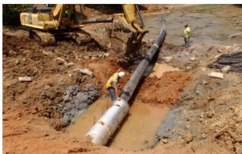
Figure 4-48: Replacement of Pipe in Dam (KRG Utility)
