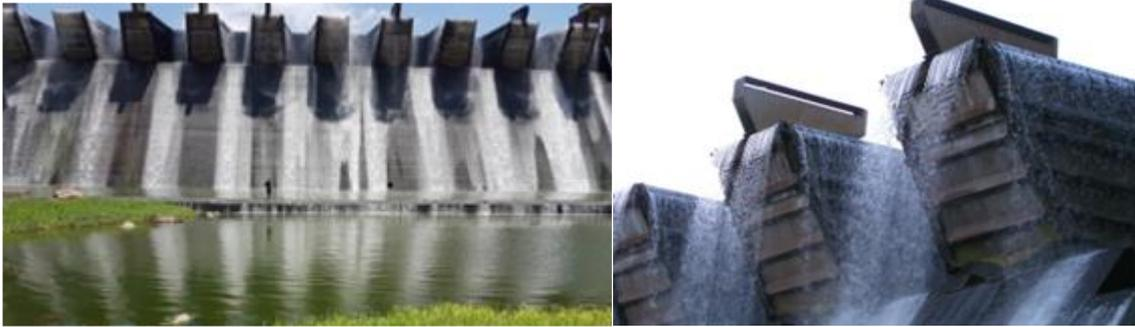
Concrete gravity dam, 32 meters high, with 92 years in operation. Service spillway was rehabilitated for increasing storage and for hydraulic safety with steel fuse gates (Hydro plus, at Erbisti). Detail shows a steel structure and well component on top.
