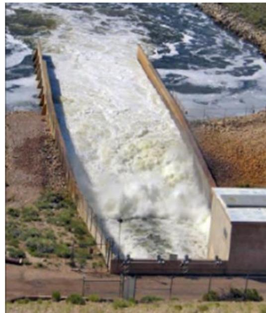
Figure 5-5: Energy dissipation by turbulence due to Hydraulic Jump (Stilling basin FEMA, 2010).
