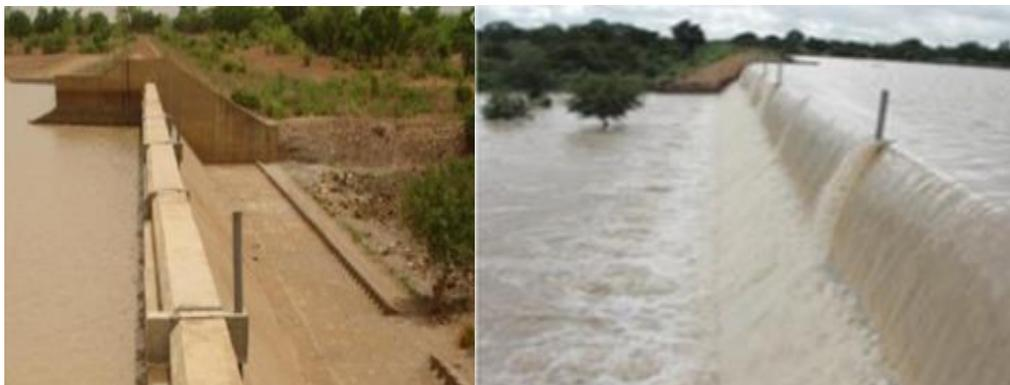
Figure 3-88: Wedbila Dam, Burkina Faso. Small embankment dam. Spillway with fuse plug con-crete blocks (HydroCoop).
