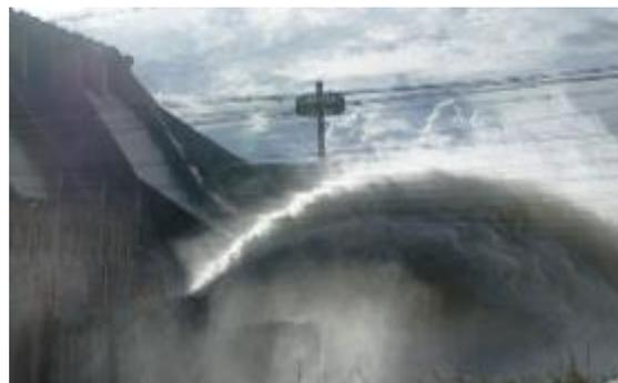
Figure 5-27: Jet trajectory and effects of dispersion and aeration, Guri dam, Venezuela (Marcano, 2000)
