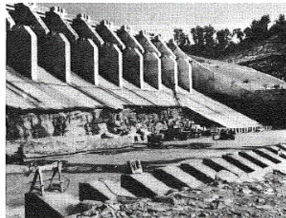
Figure 5-79: Damage due to cavitation + hydrodynamic pressure fluctuation, Karnafuli dam, Bangladesh.
