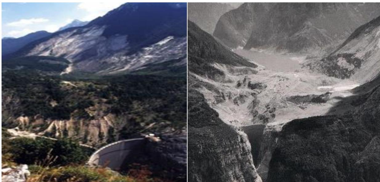
Figure 2-1: Vajont Dam and the left bank Sliding.
