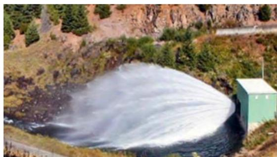
Figure 5-9: Energy dissipation by dispersion of water in air (emerging flow from a valve) (FEMA, 2010)
