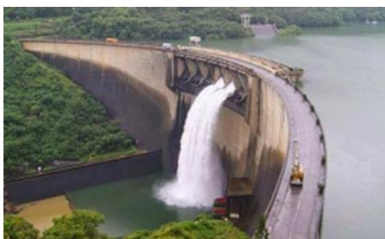
Figure 5-49: Free jet with energy dissipation at toe of Arch dam.
