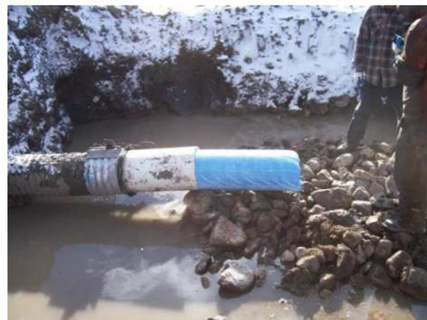
Figure 4-51: CIPP installation at Upper Taylor Dam, Powell County, Montana (Fischer 2009)
