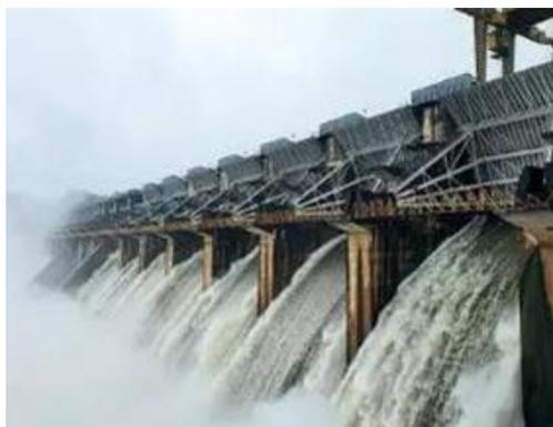
Figure 3-126: Very large spillway, 27 radial gates, 15.4 m x 14 m, 49,500 m<sup>3</sup>/s, 130 m<sup>3</sup>/s/m each bay
