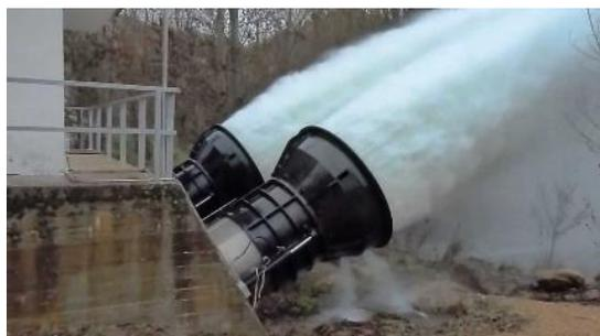
Figure 4-32: Howell Bungler Valve at Beleña Dam, Spain. (2013)
