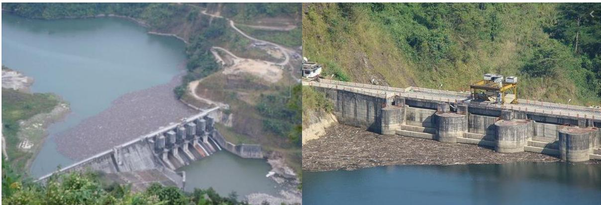
Figure 3-32: Ranaganadi dam, India.  $H = 24.3\text{m}$ ,  $q = 152 \text{ m}^3/\text{s}/\text{m}$ .
