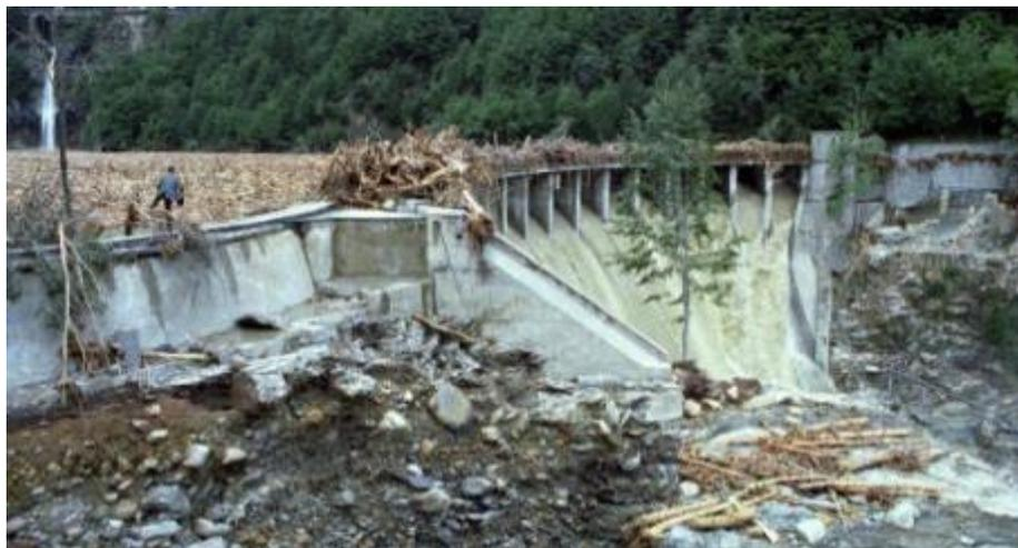
Figure 2-2: Floating debris obstructing the Palagnedra Dam spillway during the 1978 flood (Swiss Committee of Large Dams, 2017).
