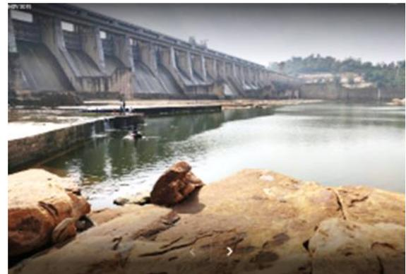
Figure 5-39: Ranapratap Sagar dam, height 53.8 m, Flip Bucket
