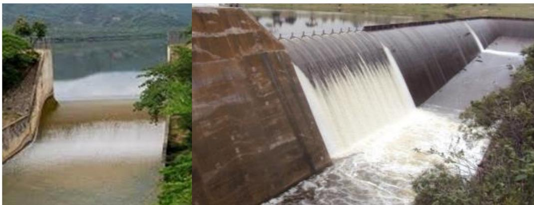
Figure 3-14: Service spillways. Control structure: free discharge, shaped crest, straight frontal and side channels.
