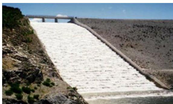
Figure 5-50: Stepped chute on RCC dam
