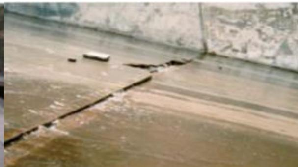
Figure 3-141: Stagnation pressure. Collapse of slab and offset in a transverse contraction joint with damages (Trojanowski, 2005)
