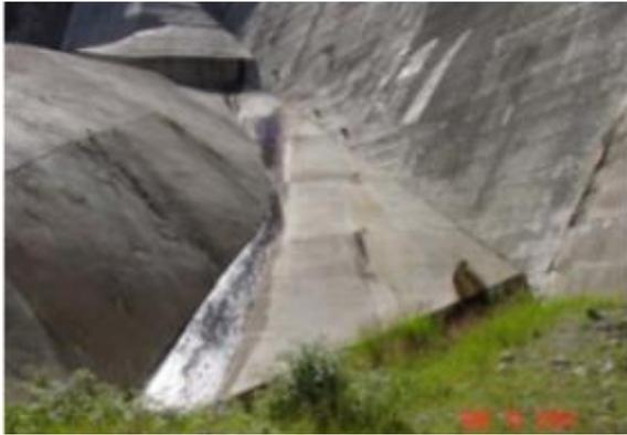
Figure 2-31: Concrete overtopping protection at the downstream toe of a dam
