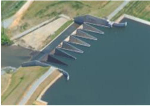
Figure 3-52: Townhead dam. Labyrinth weir with 7 cycles (Schnabel Engineering)
