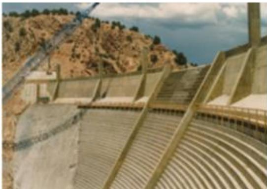
Figure 2-30: Concrete overtopping protection for Santa Cruz Dam.
