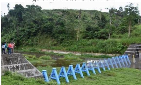
Figure 2-8: Open steel check dams for debris trapping.
