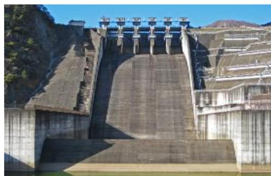
Figure 5-12: Typical stilling basin (with downstream weir to control TW)
