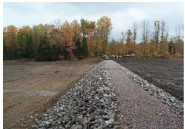
Figure 3-47: Fuse plug rebuilt. Silver Lake Dam, Dead River, Michigan, USA (FERC).
