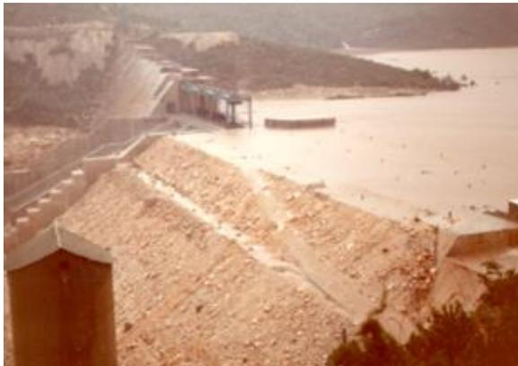
Figure 2-23: Tous Dam (Spain) failure due to overtopping in the flood of 1982.
