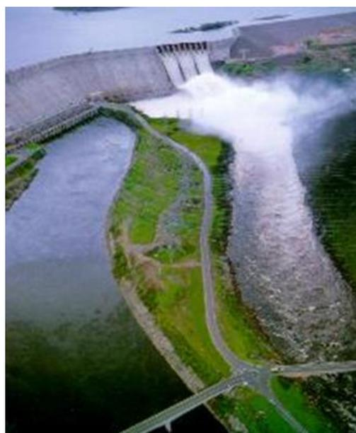
Figure 5-61: Flip bucket, plunge pool and exit channel in a high head spillway; Guri dam, Venezuela (EDELCA, 2000)
