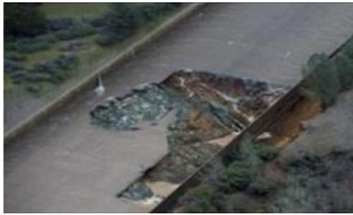
Figure 3-138: Failure of service spillway due to combine destructive processes. Oroville Dam, USA.
