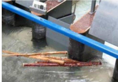
Figure 2-18: Obstruction in a three-bay system.
