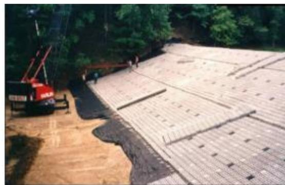
Figure 2-25: Placement of cable tied mats over a geotextile on the downstream face of Strahl Dam, Indiana, USA
