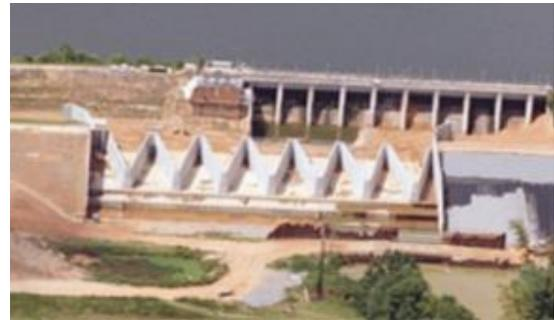
Figure 3-55: Townhead dam. Labyrinth weir. New dam located closely downstream of old dam(Schnabel Engineering)
