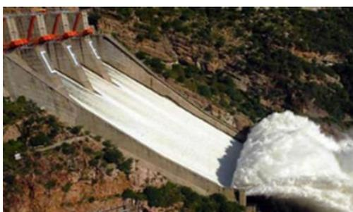
Figure 5-6: Energy dissipation by dispersion in the air and impact (flip bucket).
