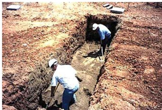
Figure 4-55: Filter diaphragm trench (NRCS Ch.45, 2007)
