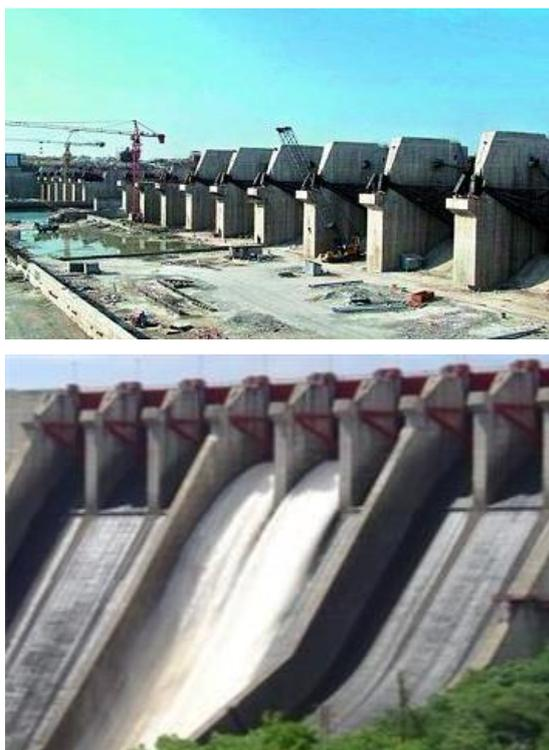
Figure 3-19: Typical shaped crested weir (Ogee) controlled with gates.
