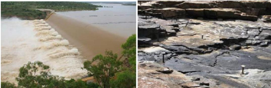
Figure 5-85: Scour of top layer of fractured rock and exposed anchors, after flood (Bollaert and Lesleighter, 2014)
