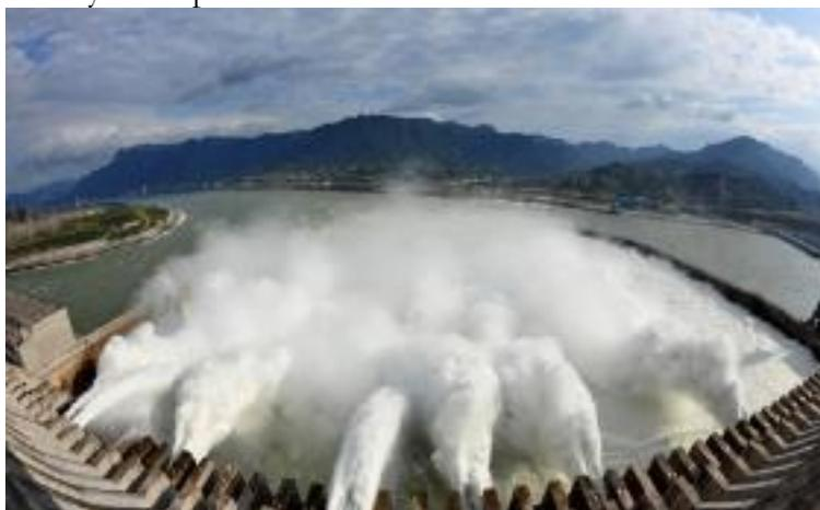
Figure 5-47: Three Gorges dam, China, bottom outlets (sluices), exit velocity of  $35 \text{ m/s}$ , (Chanson, 2015)
