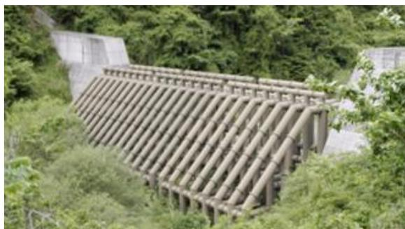
Figure 2-7: A Steel Check Dam.
