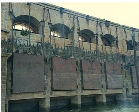
Figure 4-15: Gates in Sluice Intake at KRS, Karnataka (CWC; 2018)
