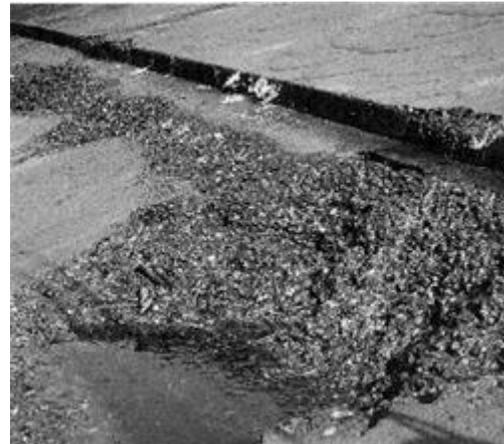
Figure 3-140: Cavitation damages, Level 4. Guri dam, Venezuela (EDELCA).
