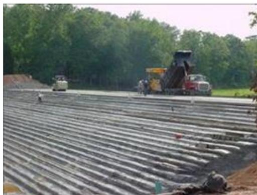
Figure 3-97: Thomaston Dam, Georgia, USA. RCC overtopping protection in entire length of dam.
