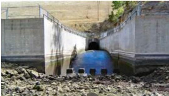
Figure 5-17: Stilling basin at the outlet of a tunnel (FEMA, 2010)
