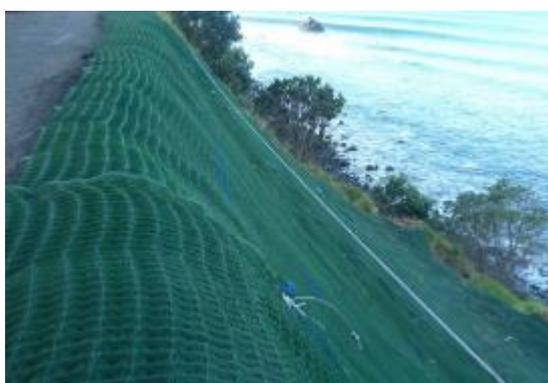
Figure 5-56: Geotechnical product with vegetation, bank protection in a natural channel
