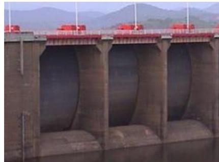
Figure 3-16: Service spillways. Controlled weir with radial gates
