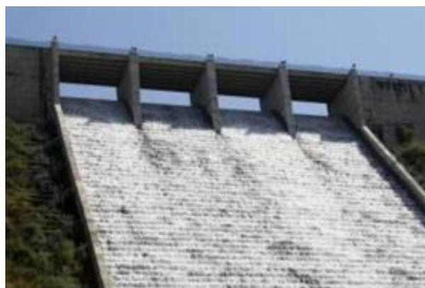
Figure 3-18: Service spillways. Steeped chutes on gravity dam (RCC).
