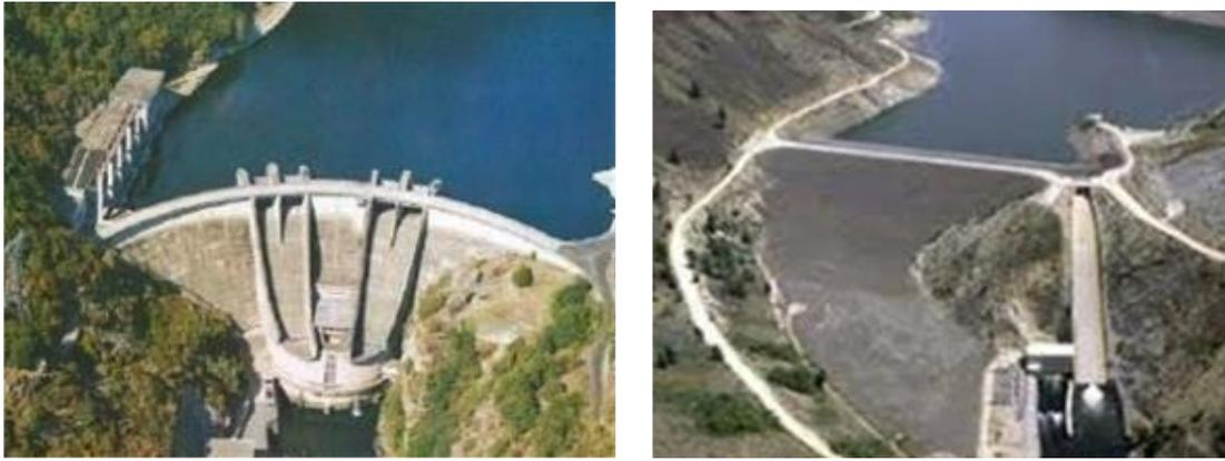
Figure 3-11: Service spillways. On a concrete gravity dam and left abutment of an embankment dam.
