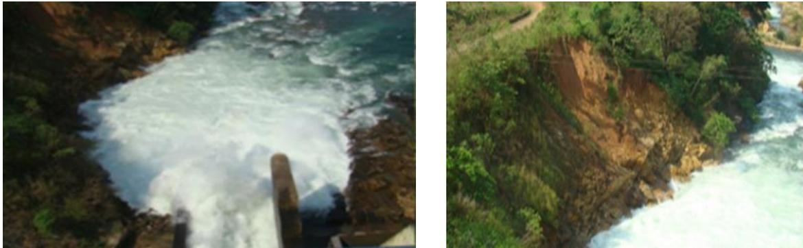
Figure 5-86: Scour of river due to bottom sluice discharge, Balimela dam, head = 30 m,  $Q= 1,135 \text{ m}^3/\text{s}$
