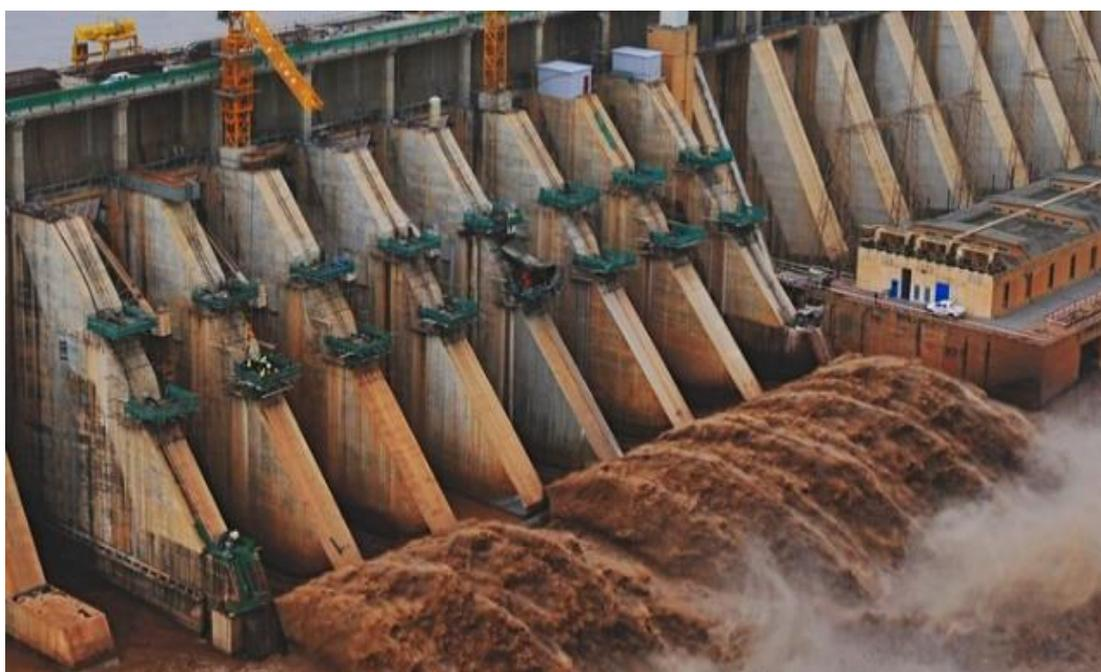
Figure 3-30: Roseires dam, Sudan. Gates 6m (H), 11.5 m (W), Q = 7,400 m<sup>3</sup>/s (SMEC)
