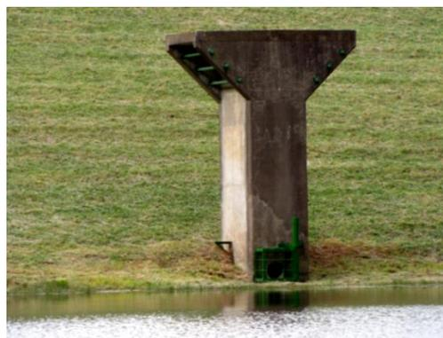
Figure 4-19: Typical riser structure (ASDSO)
