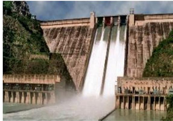
Figure 5-72: Bhakra dam, spillway and energy dissipator,  $Q = 5,587 \text{ m}^3/\text{s}$
