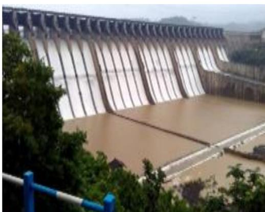
Figure 5-21: Sardar Sarovar dam, height 163 m, discharge 84,950 m<sup>3</sup>/s (Gujarat)
