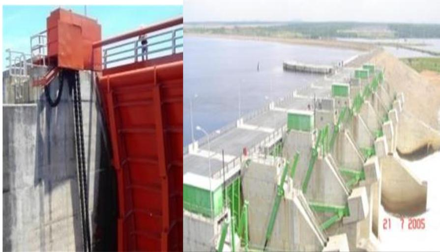
Figure 3-123: Radial gate: hoist equipment by chain and hydraulic (Guri and Caruachi Dams, on Caroni river, EDELCA, Venezuela)
