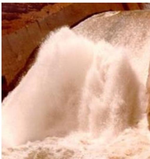
Figure 3-143: Vertical displacement of concrete slab in a chute due to hydraulic jacking (USBR)
