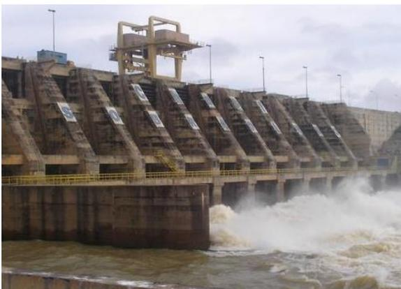
Figure 3-33: Sobradinho Hydroelectric Project Dam, Brazil, 12 gates 7.5m (H)x 9.8m (W). Heat over sill=30.2m,  $Q = 22,855 \text{ m}^3/\text{s}$ ,  $Q_{1\text{bay}} = 1,905 \text{ m}^3/\text{s}$  (Chefs)
