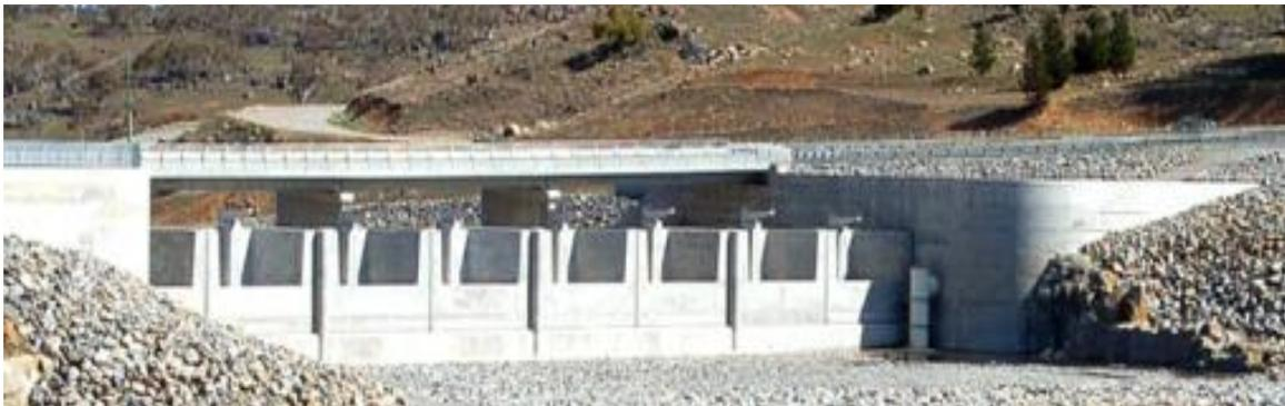
Figure 3-80: Typical fusegate installation (HydroPlus)
