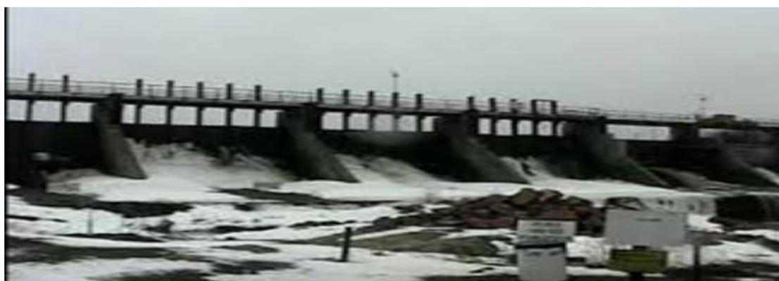
Figure 2-21: Ice accumulation in spillway
