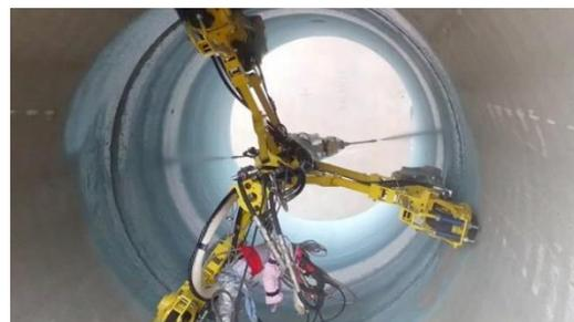
Figure 4-52: Spray lining material for conduit (D.A.V. 2020)
