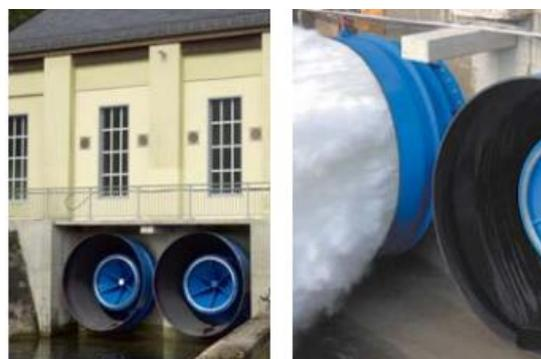
Figure 4-31: Hollow Jet Valves at Rur Dam Germany (VAG, 2016)
