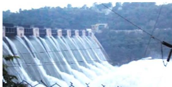
Figure 5-35: Gandhi Sagar dam, height 62 m, Flip Bucket
