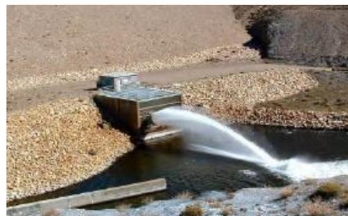
Figure 5-54: Fixed cone valve with hood and concentrated jet into a plunge pool (FEMA, 2010)
