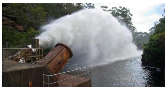
Figure 4-10: Cataract Dam outlet works discharging low flow requirements Dam (Water NSW)
