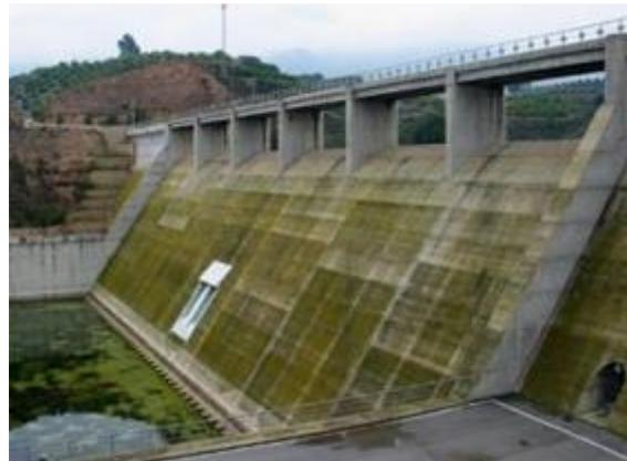
Figure 3-13: Service spillways. Control structure: free discharge, shaped crest, on concrete gravity dams.
