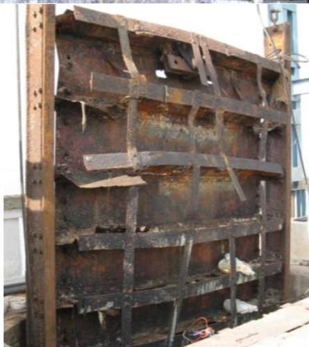
Figure 4-3: Condition of Gates in KRS Dam (CWC; 2018)
