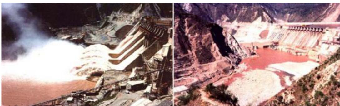
Figure 5-82: Erosion damages in river's environment. Salal dam, India (Bhajantri et al.)
