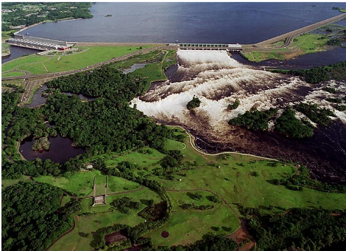
Figure B.1- 70 Macagua Spillway and flow behavior with Dyke System in operation. (Vilchez)
