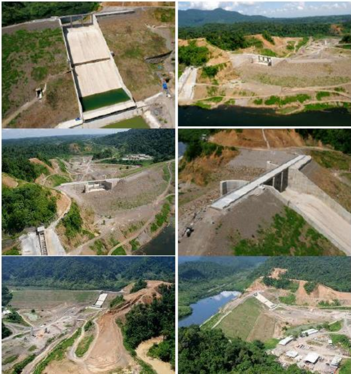
Figure B.3- 14 El Guapo Dam – after Rehabilitation. (C. Hernández, 2008)
