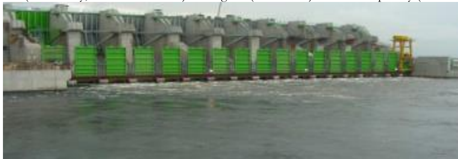
Figure B.1- 74 Caruachi Hydroelectric Project - Double Body Spillway during construction; 18 no., 9m x 5.5m sluices (lower body, for river diversion) and 9 gates (15.24x21m) for service spillway (EDELCA)
