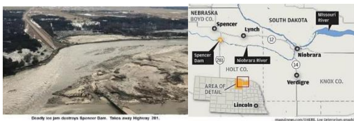
Figure B4- 4 The ice jam took away Highway-281 bridge. Location map of the Spencer dam (maps4news.com).
