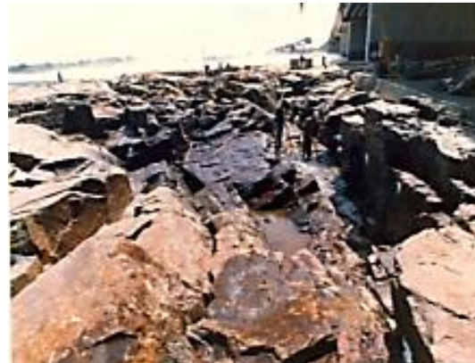
Figure B.1- 57 Macagua Spillway rehabilitation works. Cleaning geologically weak areas in front of the spillway. (EDELCA)
