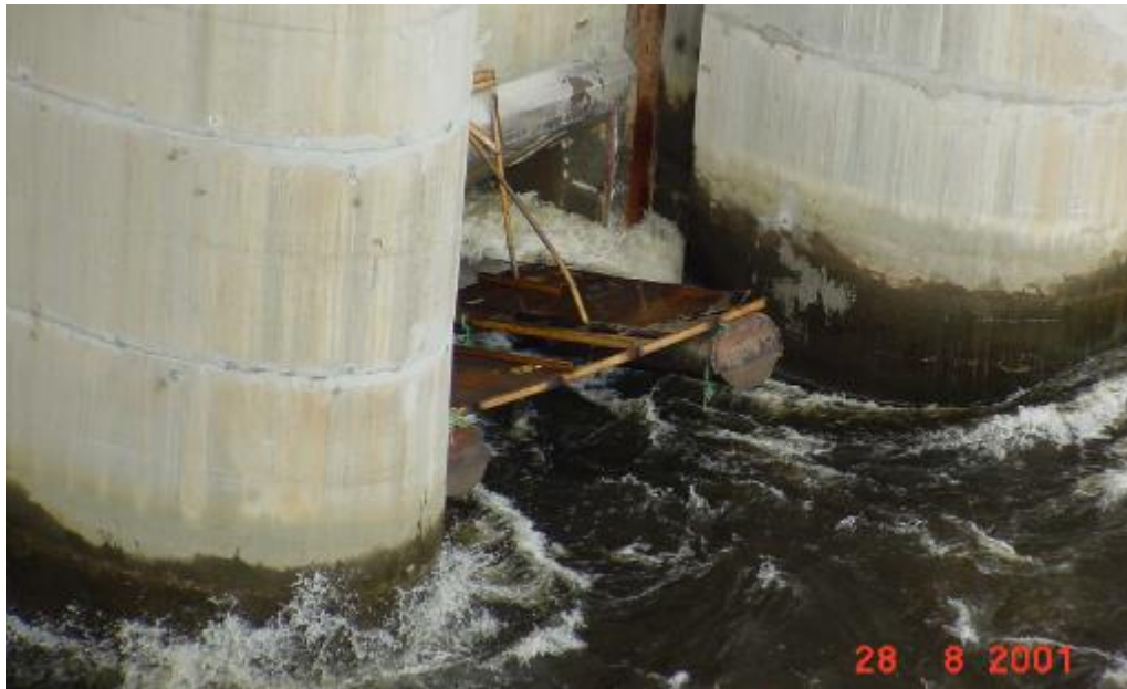
Figure C- 8 Precarious Mining Barge creating an emergency in a dam without retention system, Caruachi Project, Venezuela.
