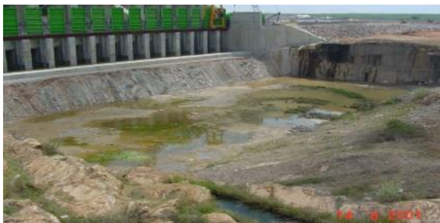
Figure B.1- 77 Caruachi Hydroelectric Project –Spillway pre excavated plunge pool. (EDELCA)
