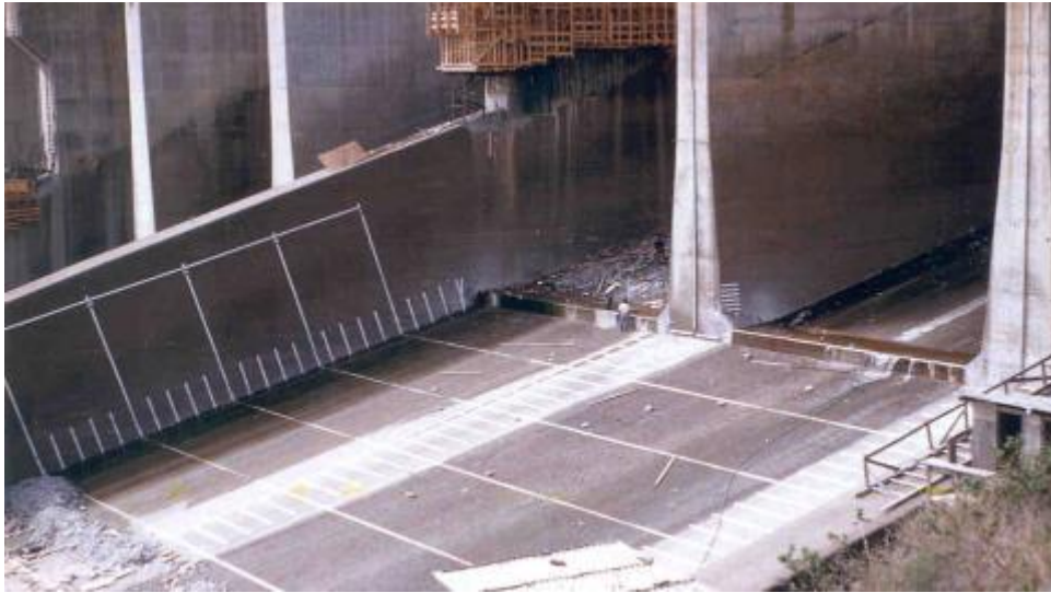
Figure B.1- 27 Prototype ramp 0.75 m, 17° exit angle built in the 3 bays of original Chute system of measurement of the Cavity length and piezometric taps. (EDELCA)
