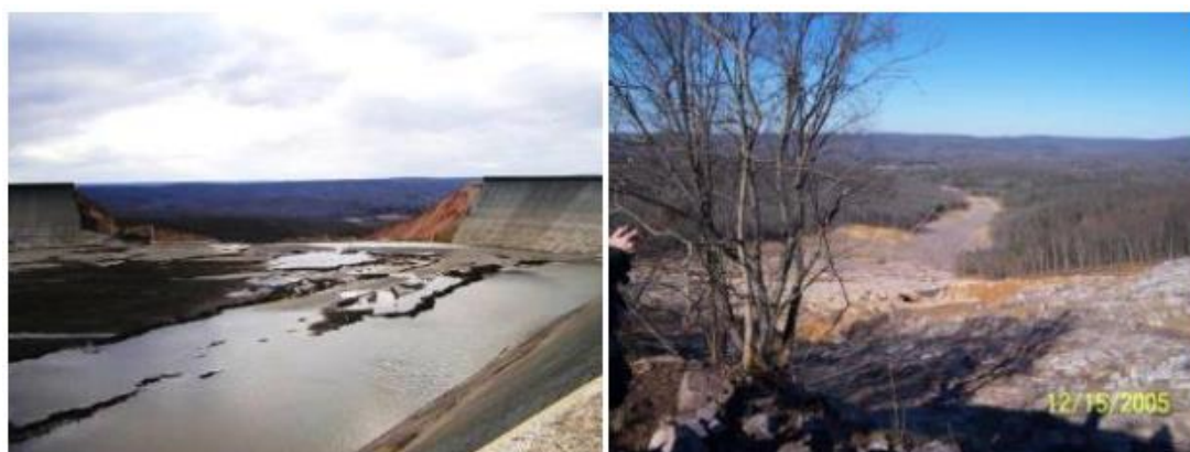
Figure B.2- 3 A large section of the upper reservoir failed, draining over a billion gallons of water in less than half an hour (left) and the flood path downstream of the breach section (right).
