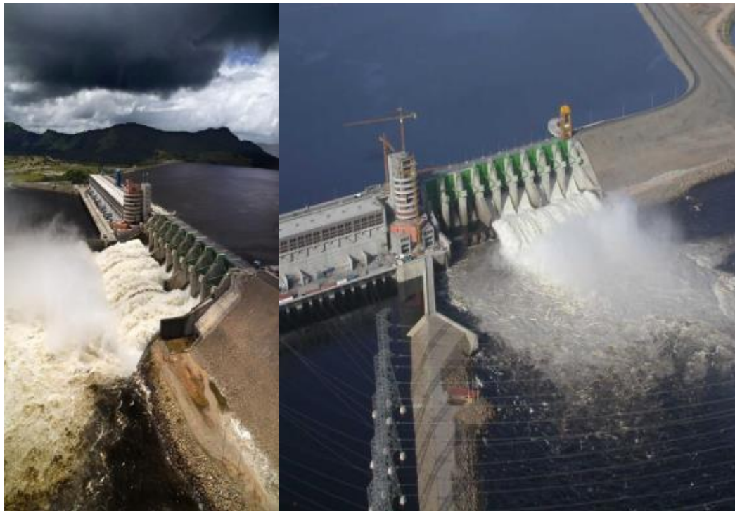
Figure B.1- 76 Caruachi Hydroelectric Project- Surface spillway operating. Note jet being thrown very close to the structure and apparent good energy dissipation downstream of the impact zone. (EDELCA)
