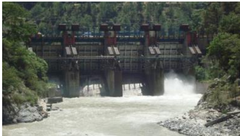
Figure B.5- 1 Downstream view of Maneri Dam. (CWC)
