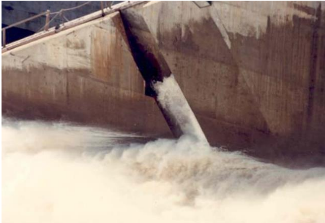
Figure B.1- 48 Chute 3 Final Stage of Guri Spillway. Lower aerator in operation. (EDELCA)
