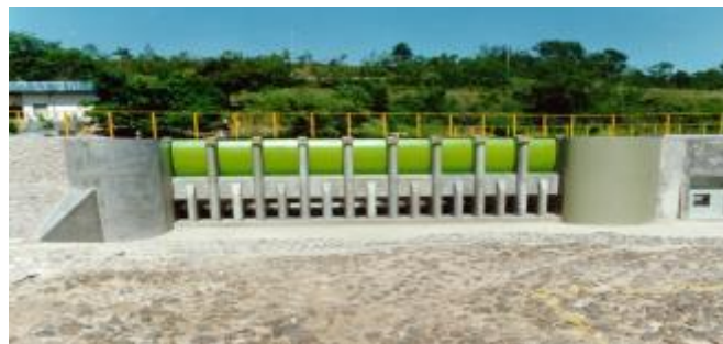
Figure B.1- 83 Caruachi Hydroelectric Project –Comprehensive 3D Physical Model Scale 1.80. View of double body spillway from upstream. (Marcano, 2002)
