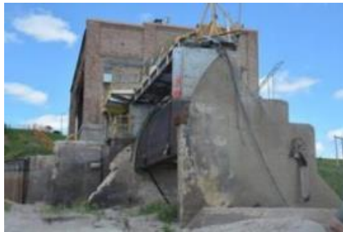
Figure B4- 11 Looking north back towards the powerhouse of the Spencer Dam, 2019.
