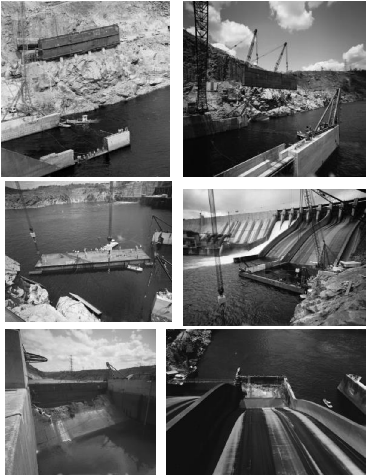
Figure B.1- 10 Process of placing the floating bulkhead to initiate the repair works. (EDELCA)
