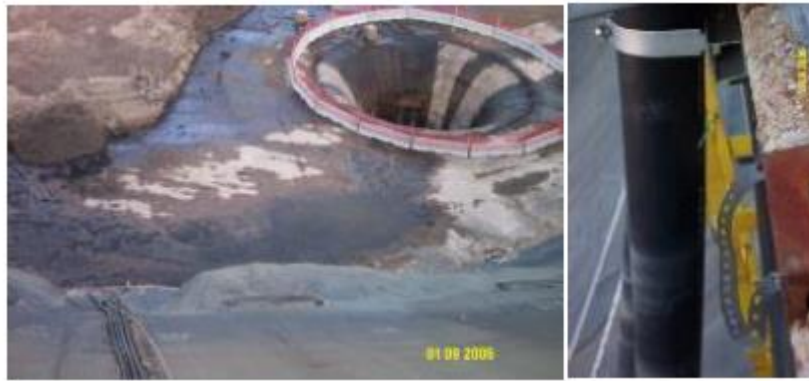
Figure B.2- 12 Instrumentation location relative to the water conveyance shaft (left) and high-water marks on HDPE Tubes, (Courtesy of Missouri DNR)
