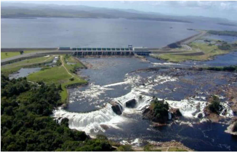
Figure B.1- 68 The Falls operating with the Dykes system operating for ecological flows. (Routes.global)
