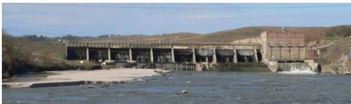
Figure B4- 5 The Spencer dam and the powerhouse before failure (looking upstream).
