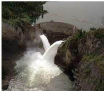
Figure D-38 Spillways in operation.
