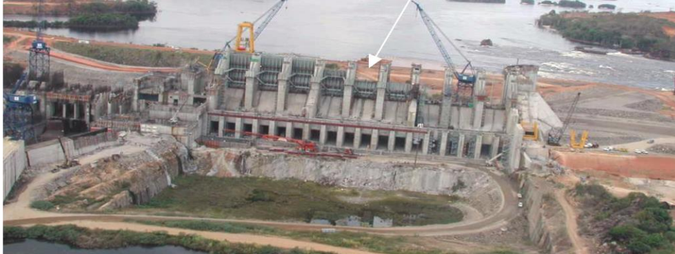
Figure B.1- 74 Caruachi Hydroelectric Project - Double Body Spillway during construction; 18 no., 9m x 5.5m sluices (lower body, for river diversion) and 9 gates (15.24x21m) for service spillway (EDELCA)
