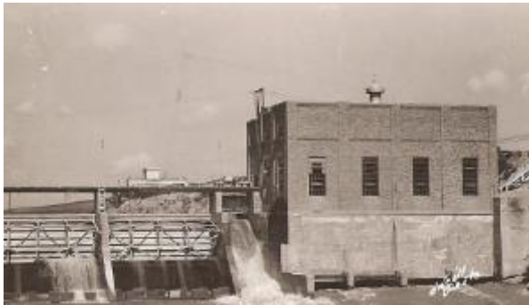
Figure B4- 6 Spencer Dam as it appears in its rebuilt condition in 1945, after a 1936 failure of the dam's overflow weir, 1945.
