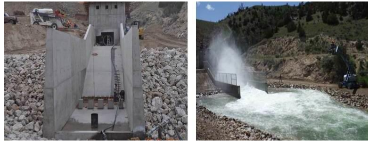
Figure D- 71 Ruby Dam outlet works under construction and operational testing.
