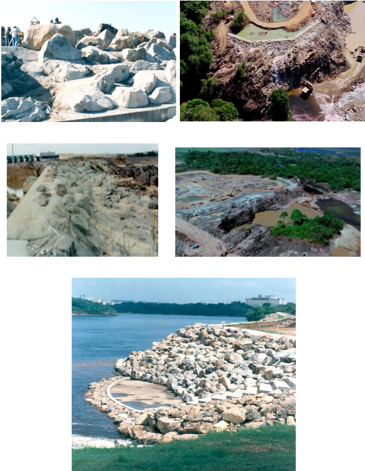
Figure B.1- 67 Rehabilitation works to restore the flow distribution to La Llovizna Falls. (EDELCA)
