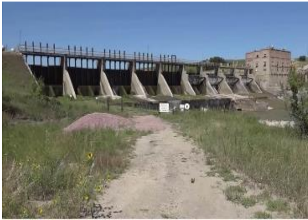
Figure B4- 1 The pre-failure Spencer dam.
