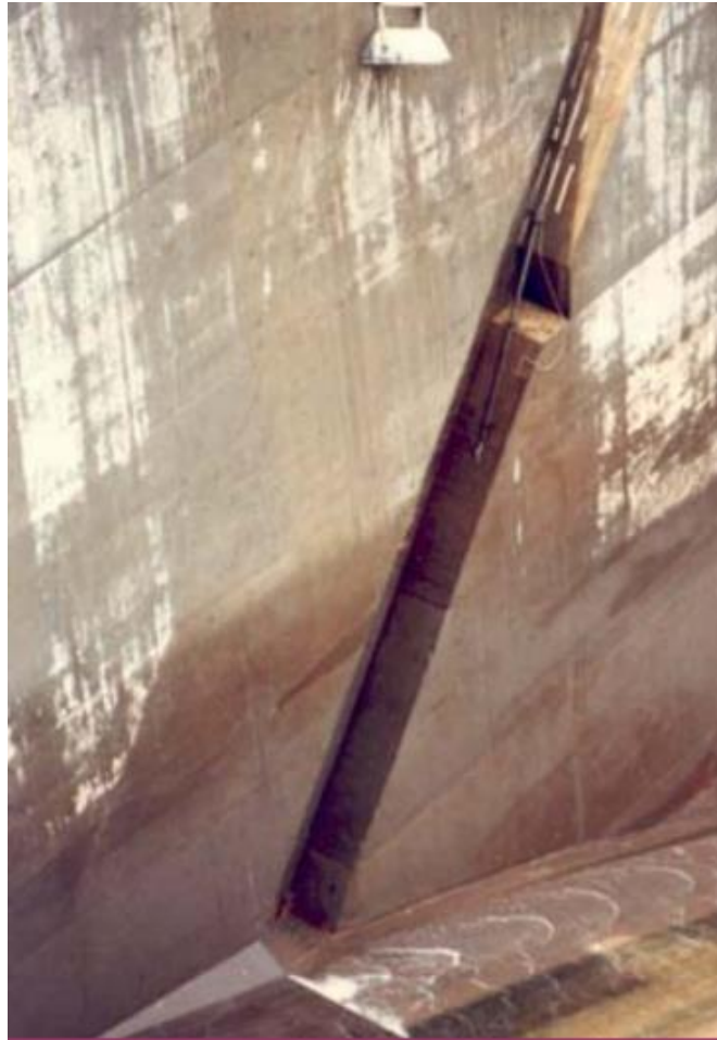
Figure B.1- 46 Chute 3 Final Stage. Lower aerator. Note the ramp, the step, the lateral ramp and the wedge. (EDELCA, 1987)
