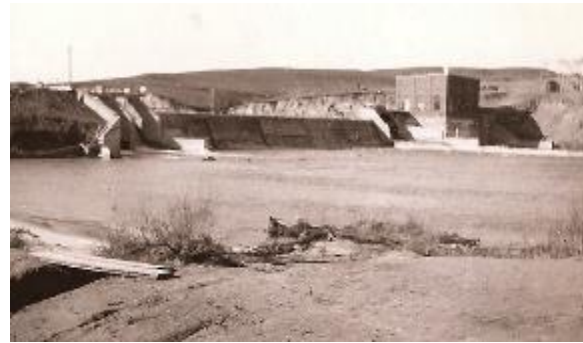
Figure B4- 7 Spencer dam soon after it was built around 1927.
