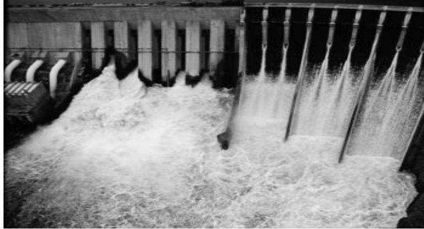
Figure B.1- 5 Diversion Sluices working together with the 3 Spillways chutes while generation has started in the first units of Power house 1. (EDELCA)
