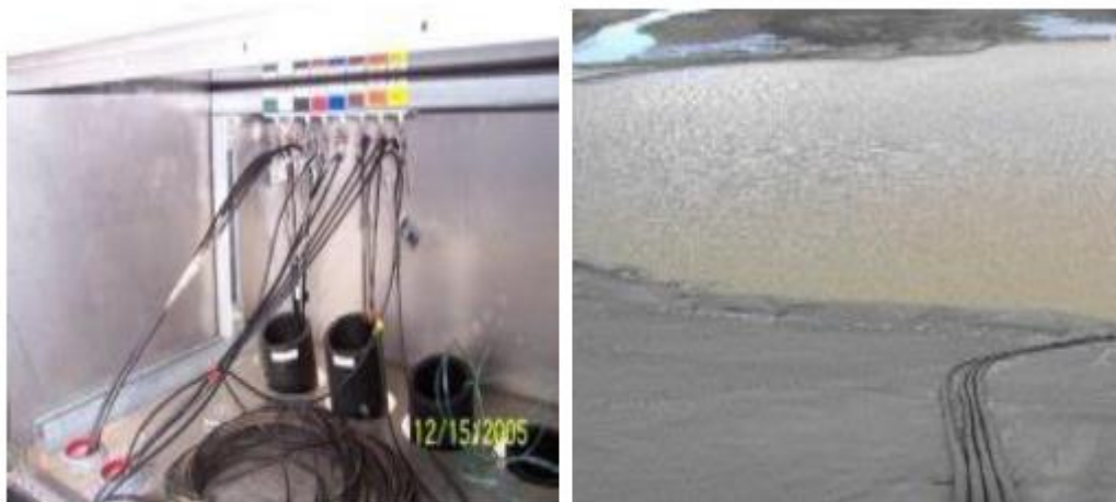
Figure B.2- 11 Cabinet containing the Duck pressure transducer and Warrick conductivity sensor wiring (left) and Bowing of HDPE Tube position on December 15, 2005 (Courtesy of Missouri DNR)
