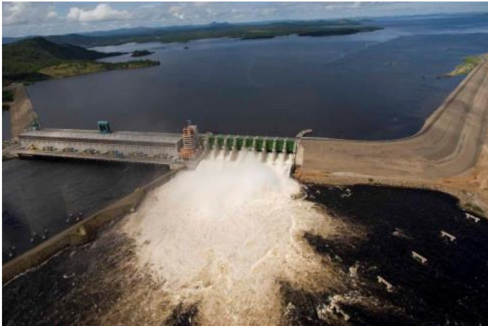
Figure B.1- 71 2,196 MW Caruachi Hydroelectric Project in the Lower Caroni, Venezuela (EDELCA)
