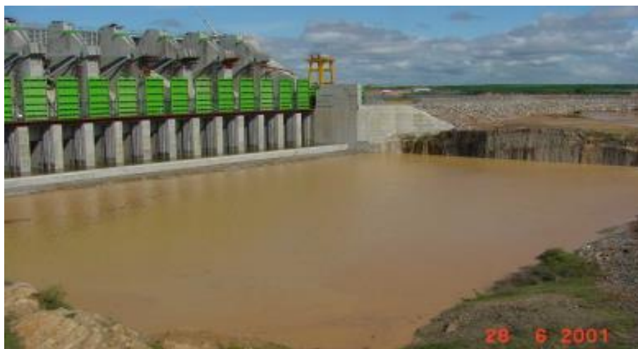
Figure B.1- 80 Caruachi Hydroelectric project. Plunge pool during first filling. (EDELCA)
