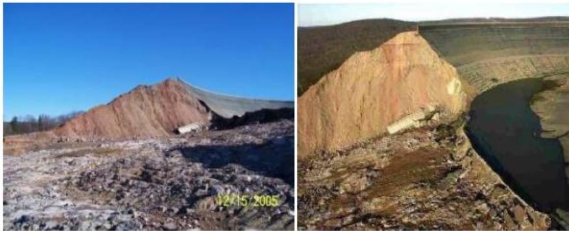
Figure B.2- 13 Weathered rock and discontinuous clay seam foundation just downstream of fish-pond area
