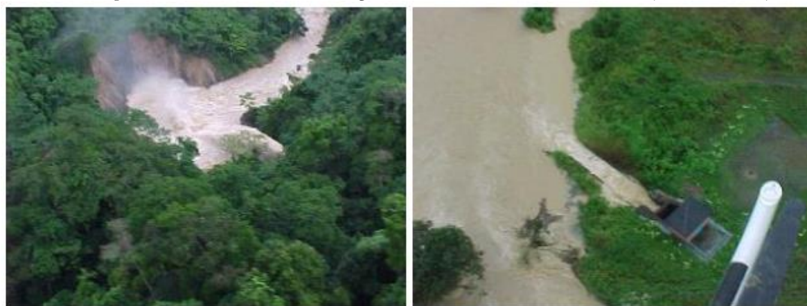
Figure B.3- 9 Secondary spillway discharge bottom outlet El Guapo Dam – December 16th, 1999. (Hidroven, 2000)
