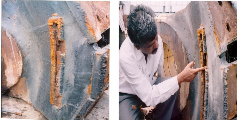
Figure B.6- 6 Spillway gate No 5 - Tie beam right side weld joint. (CWC)
