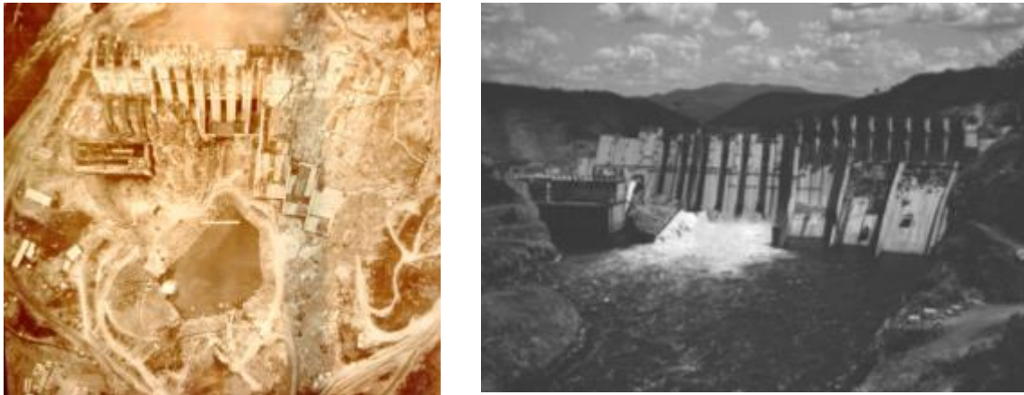
Figure B.1- 4 Left -Construction of the original works, Right - Spillway under construction. (EDELCA)
