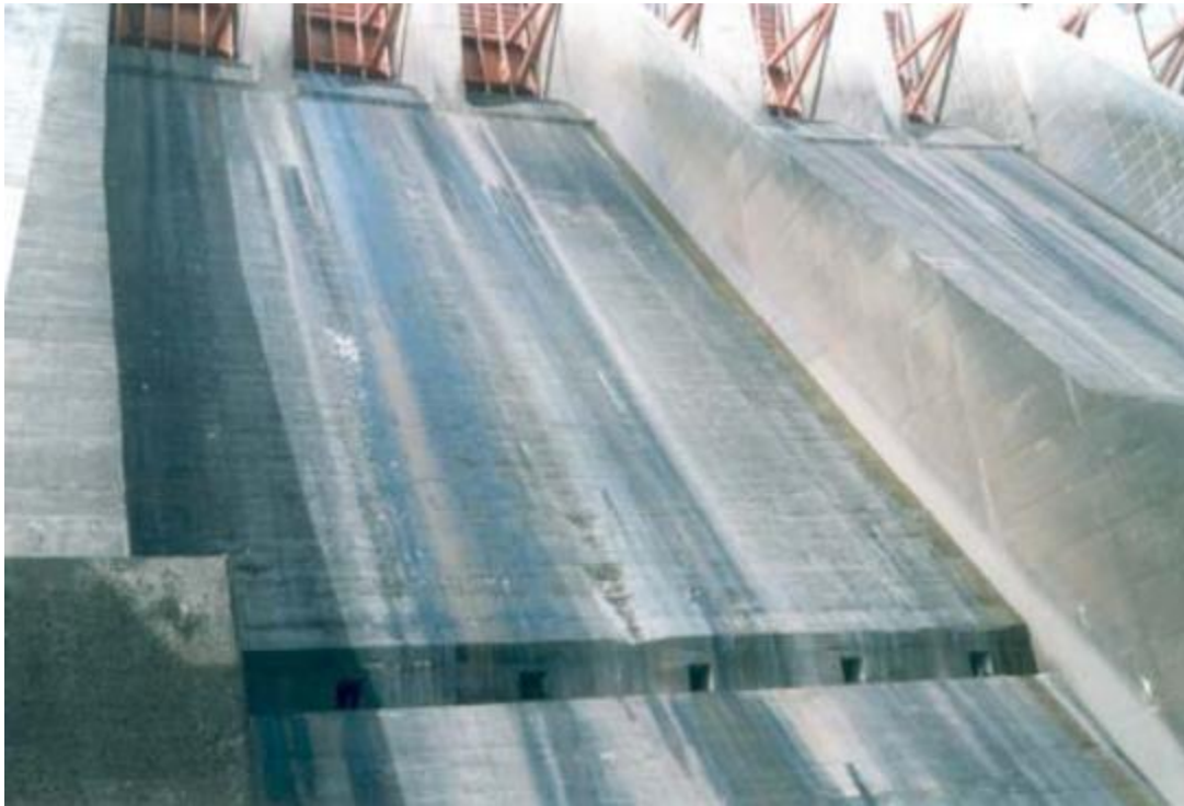
Figure B.1- 44 Chute 1 Final Stage. Lower and upper aerators. The airports, the step and the small ramp on the step in the lower aerator can be seen. The upper aerator is also visible. (EDELCA)
