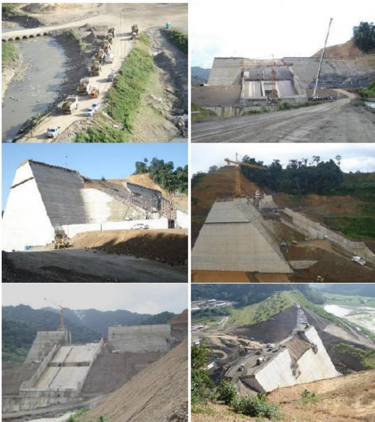
Figure B.3- 13 El Guapo Dam – Reconstruction Process. (Camargo Correa, 2005-2008).
