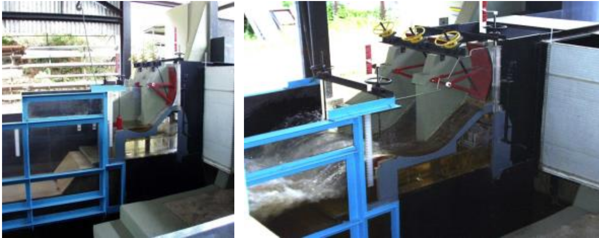
Figure B.1- 84 Caruachi Hydroelectric Project- Surface service spillway with flip bucket and pre excavated plunge pool. (Marcano, 2002)
