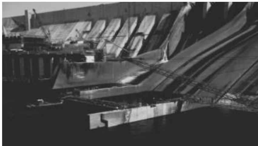
Figure B.1- 6 Walls at flip bucket locations, note that flip buckets lips are submerged (EDELCA)
