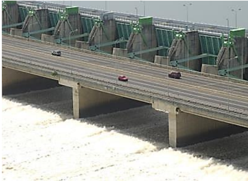
Figure B.1- 56 Spillway and 8 lane national road. (EDELCA)
