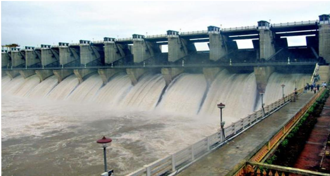
Figure B.6- 1 Narayanpur Dam Spillway in Operation. (CWC)
