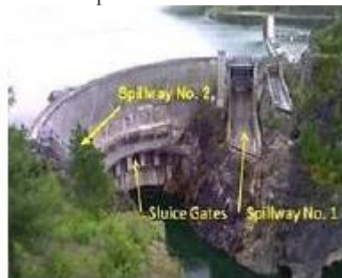
Figure D- 40 Downstream view of Boundary Dam
