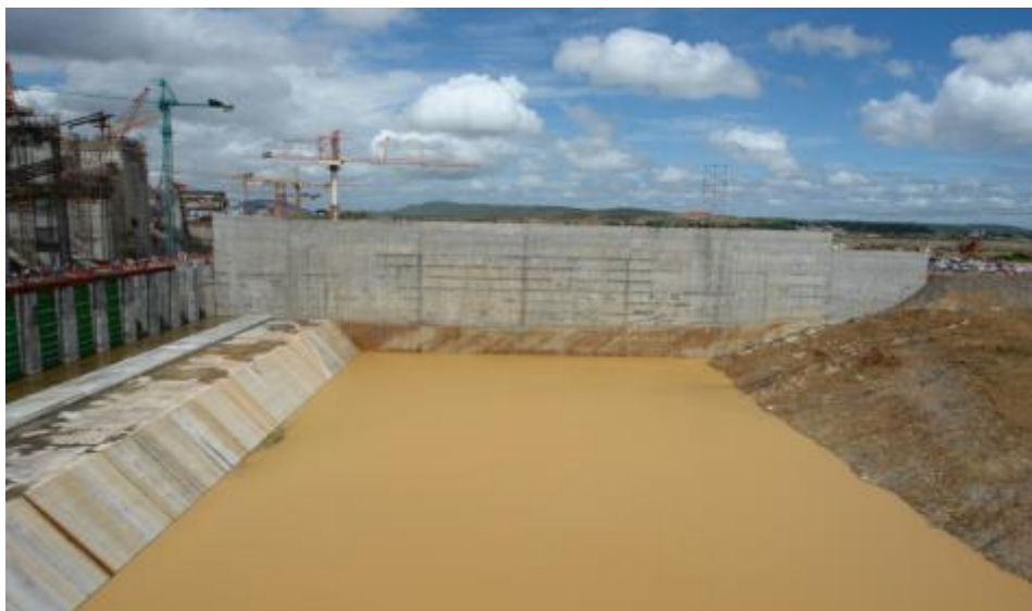
Figure B.1- 89 lateral view of concrete slab on the upstream slope of Tocomá Pre excavated Plunge pool and a wall built on the left bank of the spillway to separate flows from the Powerhouse from flows from the spillway. (CORPOELEC)
