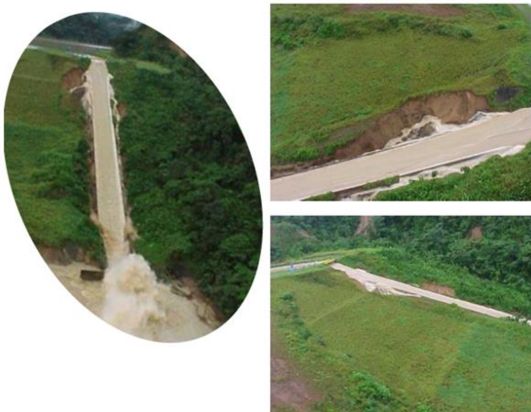
Figure B.3- 7 El Guapo Dam Chute – December 16th, 1999. (Hidroven, 2000)
