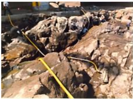
Figure B.1- 57 Macagua Spillway rehabilitation works. Cleaning geologically weak areas in front of the spillway. (EDELCA)
