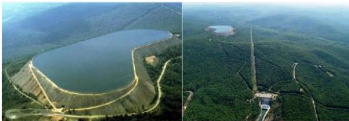
Figure B.2- 5 A view of upper reservoir (left) and powerhouse in relation to reservoir (right).
