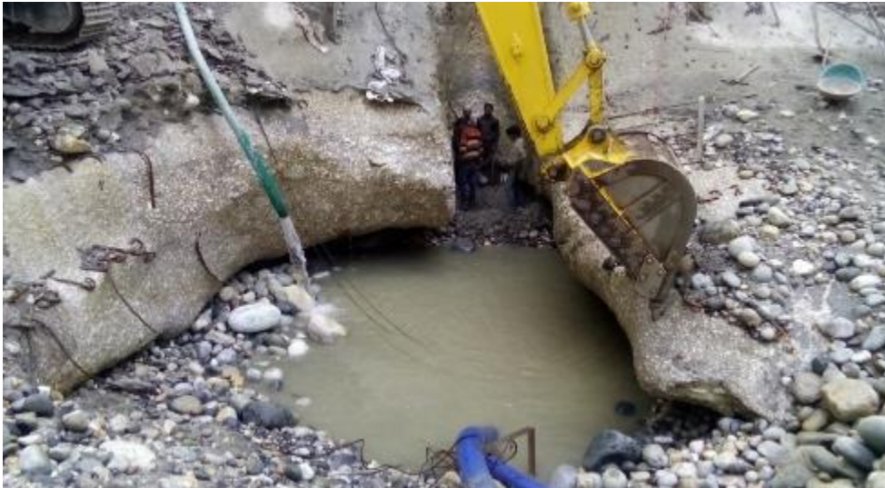
Figure B.5- 7 Cavity in Slotted Roller Bucket (CWC, 2017)
