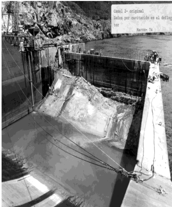
Figure B.1- 7 Repairing works in flip bucket of Chute 2 with the floating bulkhead keeping the flip buckets dry.(EDELCA)
