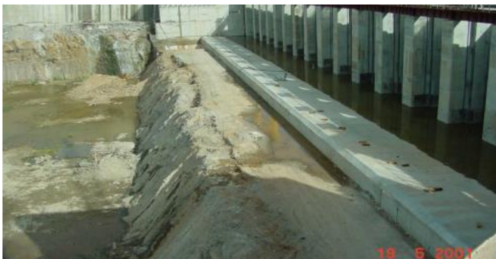
Figure B.1- 79 Short concrete slab anchored to the rock to receive the flow from the sluice at the diversion stage. Flow from the permanent spillway falls from the flip bucket into the plunge pool constructed in granitic gneiss. (EDELCA)
