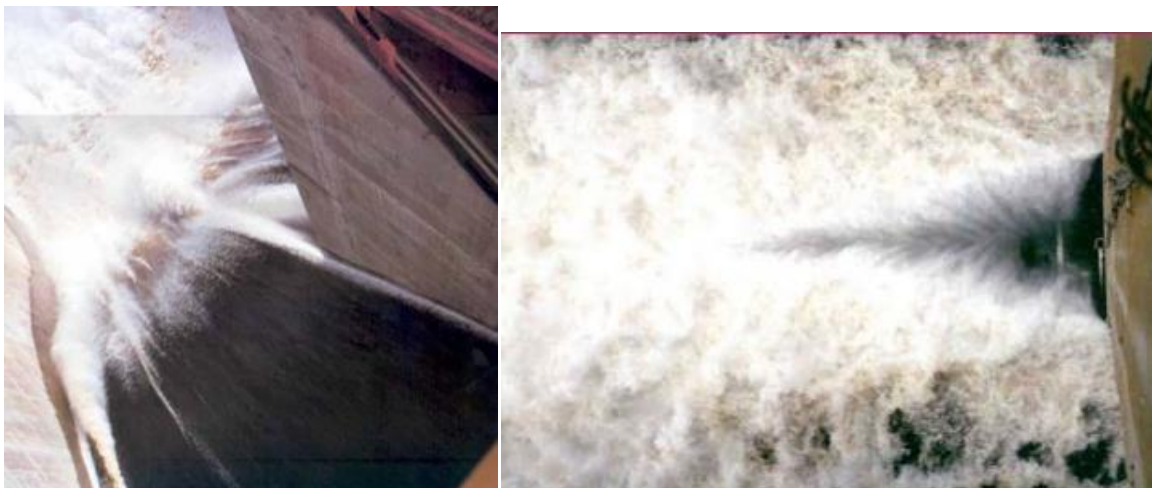
Figure B.1- 41 Guri Final Stage spillway. Upper aerator. Air intake at the rear of piers (EDELCA, 1987)
