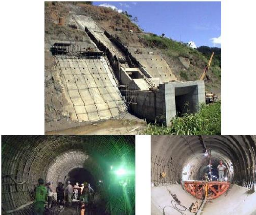
Figure B.3- 12 Bypass Tunnel El Guapo Dam (Dell'Aqua C.A., 2003).
