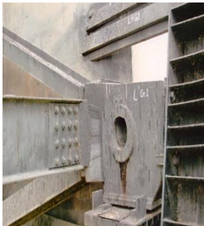
Figure B.6- 3 Typical tie beam joint. (CWC)
