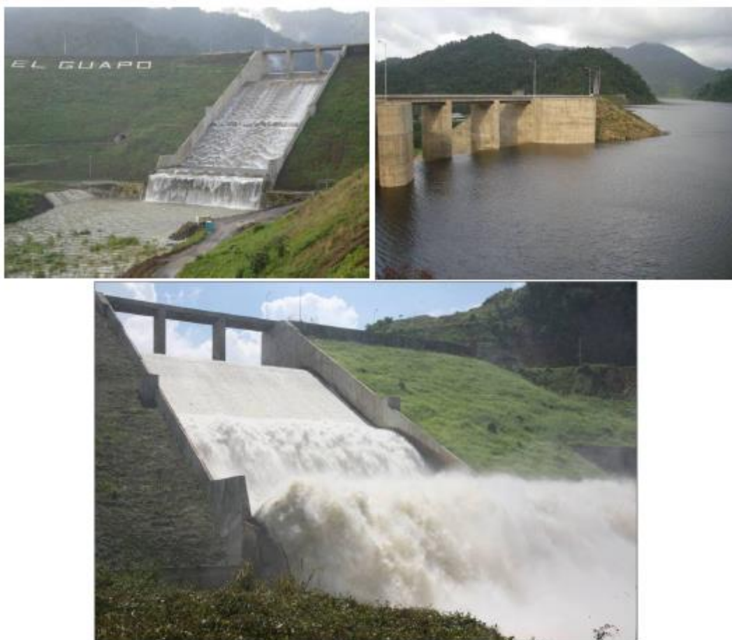
Figure B.3- 15 El Guapo Dam – operation after rehabilitation. (Camargo Correa, 2009)
