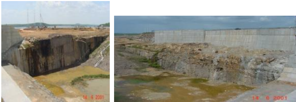
Figure B.1- 78 Left and right sides of the pre excavated plunge pool. (EDELCA)
