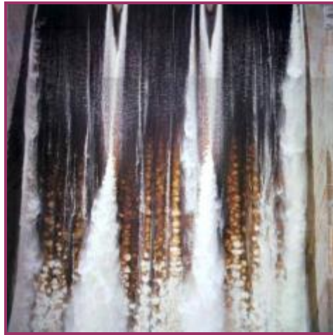
Figure B.1- 42 Flow from the upper aerator, See the air emerging from the air cavity once air flow is entrained at the rear of the gate piers (EDELCA, 1987)
