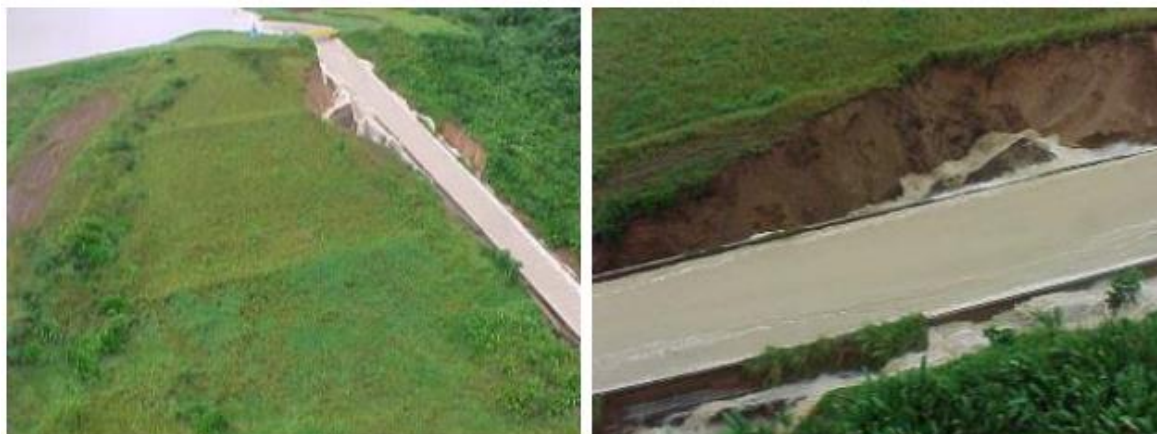
Figure B.3- 8 More Views of El Guapo Dam Chute – December 16th, 1999. (Hidroven, 2000)
