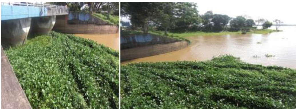
Figure C- 3 Process of flushing of Water Hyacinth by gate operation (Orinoco River Delta, Venezuela)
