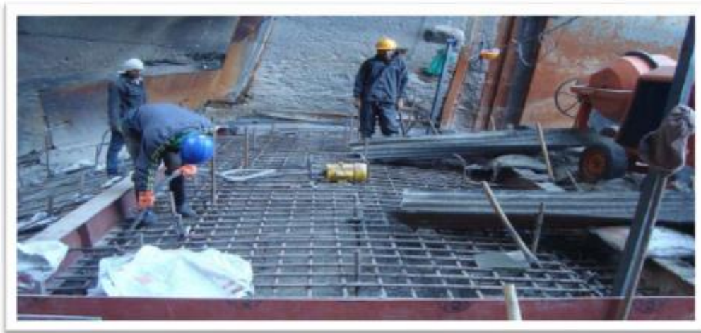
Figure B.5- 4 Laying concrete in spillway bay no 2.
