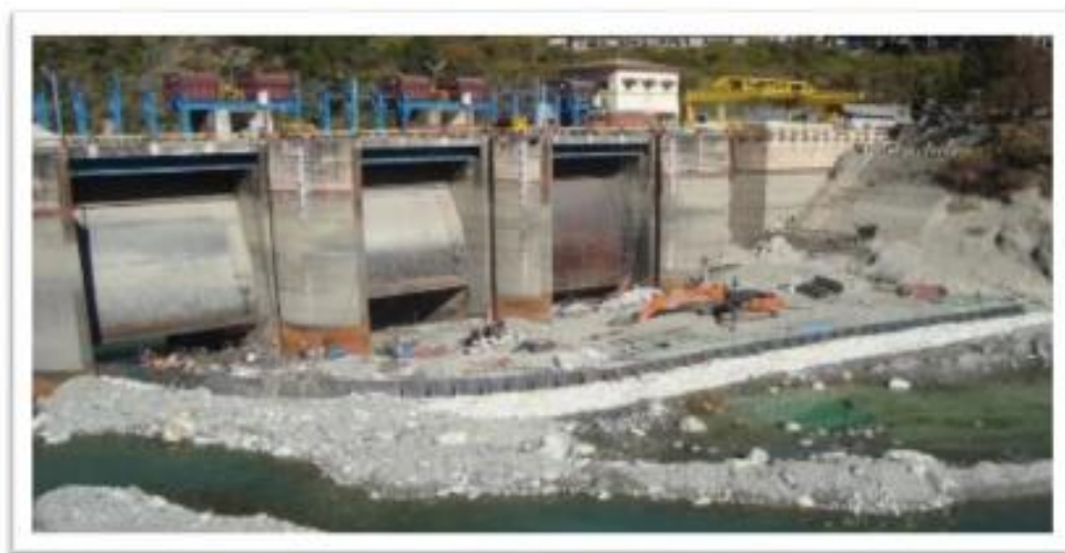
Figure B.5- 3 Temporary Bund for channelization of stream water
