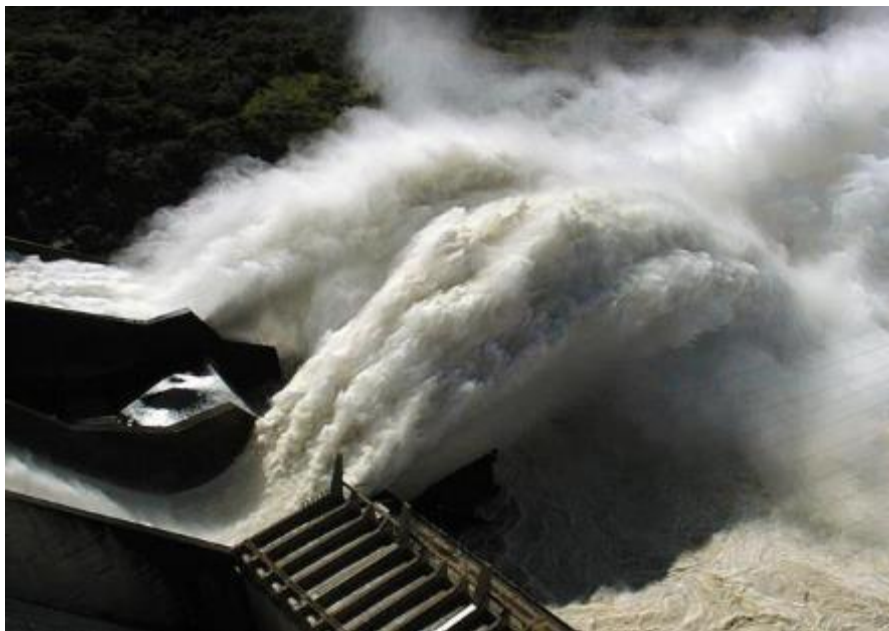
Figure B.1- 25 Chutes 1 and 3 of Guri Final Stage Spillway operating (EDELCA)
