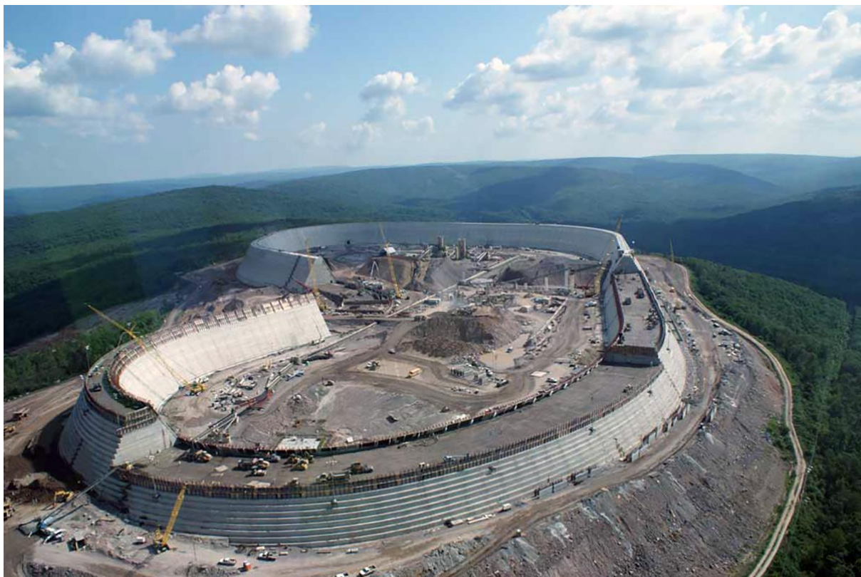
Figure B.2- 9 Reconstruction process of Taum Sauk dam with new design (gotops.com, 2010)
