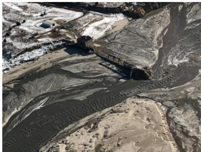
Figure B4- 3 Overwhelming ice and water breached the Spencer Dam at 5:30 am, 2019.
