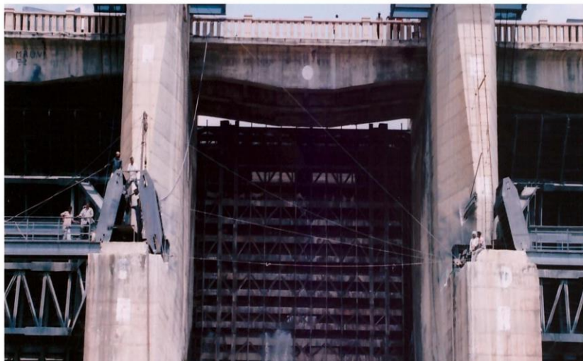
Figure B.6- 2 Stop logs placed in Bay 5 of Narayanpur Spillway after the failure. (CWC)
