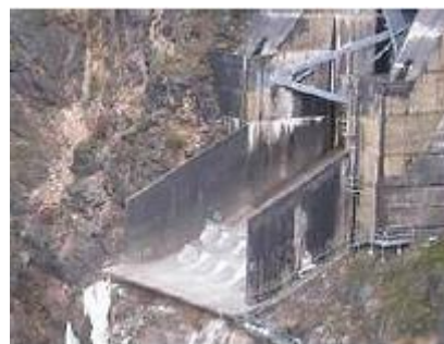
Figure D- 41 Spillway no.2 with roughness elements.
