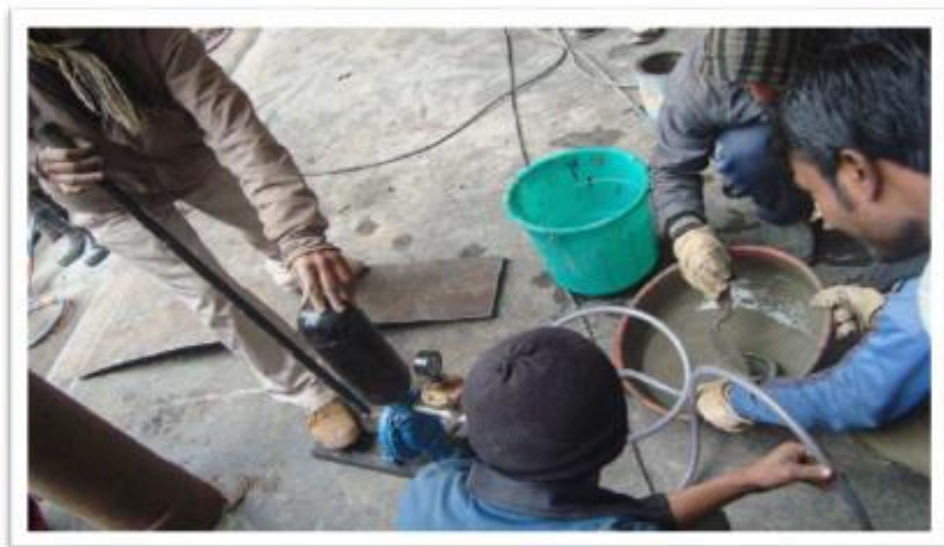
Figure B.5- 5 Laying and Grouting of MS Plate in Spillway bay no 2.
