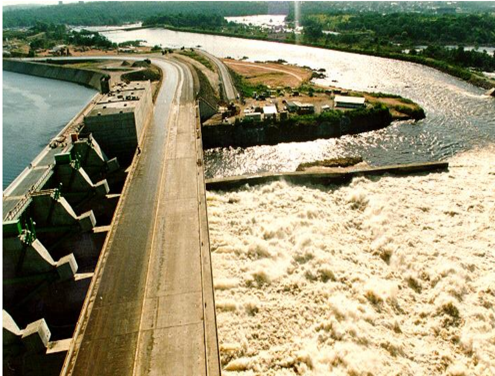
Figure B.1- 61 Macagua spillway operating with the extended concrete slab for 14,000 \text{ m}^3/\text{s} , 45% of the design spillway flow. (EDELCA)
