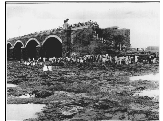
Machu II Dam failure
