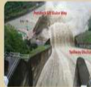
Simultaneous operation of spillway and penstock sluice venting turbid density current
