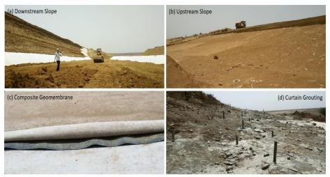
CWC redesigned the rehabilitation of the dam and used first time Geomembrane and geotextile in an earthen dam for its rehabilitation. The Rehabilitated dam got filled in 2022
