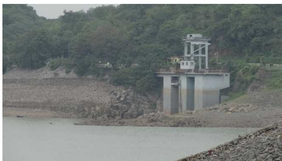
Intake tower for power generation which is one of the key assets for managing the dam.
