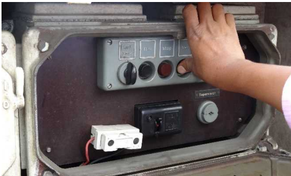
Switch box for gate operation at field
