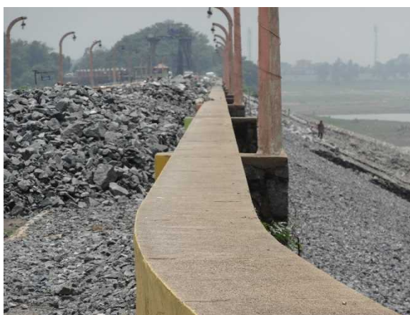
Parapet wall on left side earth dam: if sever deformation such as significant settlement or slope failure would happen; some change could be observed in this view.
