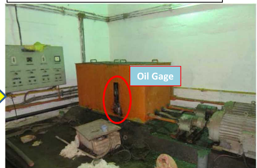
Hoist(opening and closing) equipment
