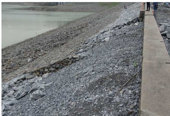
Under renovation of riprap financed by DRIP.
