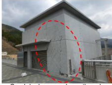
Crack by large-scale earthquake
