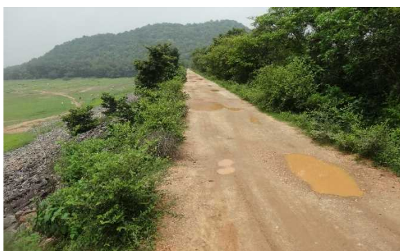
Saddle dam on left bank; the downstream slope is mostly covered with vegetation. It was recognized by DVC that cutting and clearing vegetation is necessary for appropriate maintenance. However, consultation with the forest authority is required to build the consensus.
