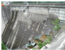
Leakage through dam body
